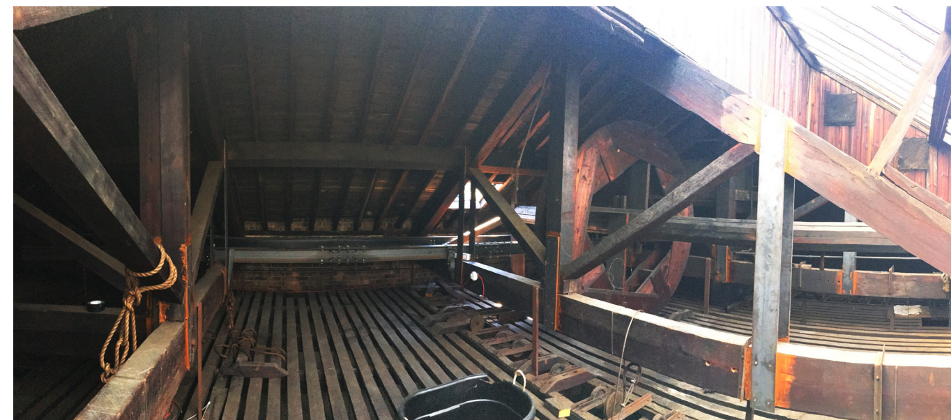
Photo of existing flytower roof structure
