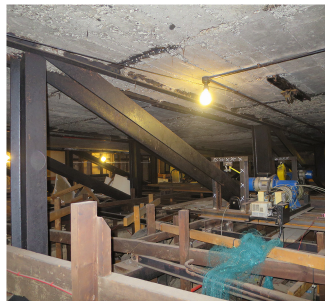
Existing roof structure over KOKO auditorium
