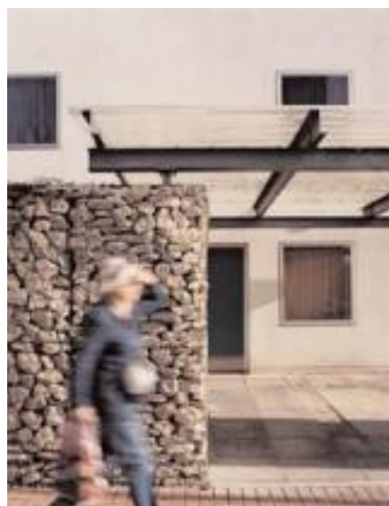
The detailing is thoughtful and responsive. The dry-stone wall at the front of the development provides visual interest and maintains the street frontage.
