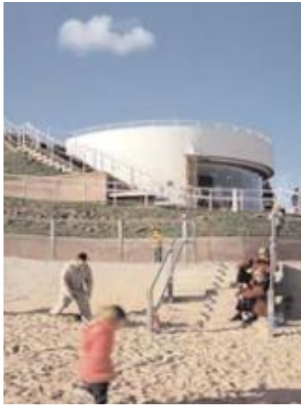
The new headland café provides a clear focal point for seafront activity.
