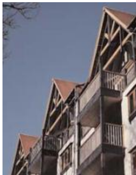
The open gables overlooking Grosvenor Park offer a modern reinterpretation of architectural details familiar from Chester's famous Rows.
