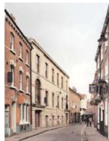
At the rear of the site, on Little Stonegate, a former chapel has been carefully restored.
