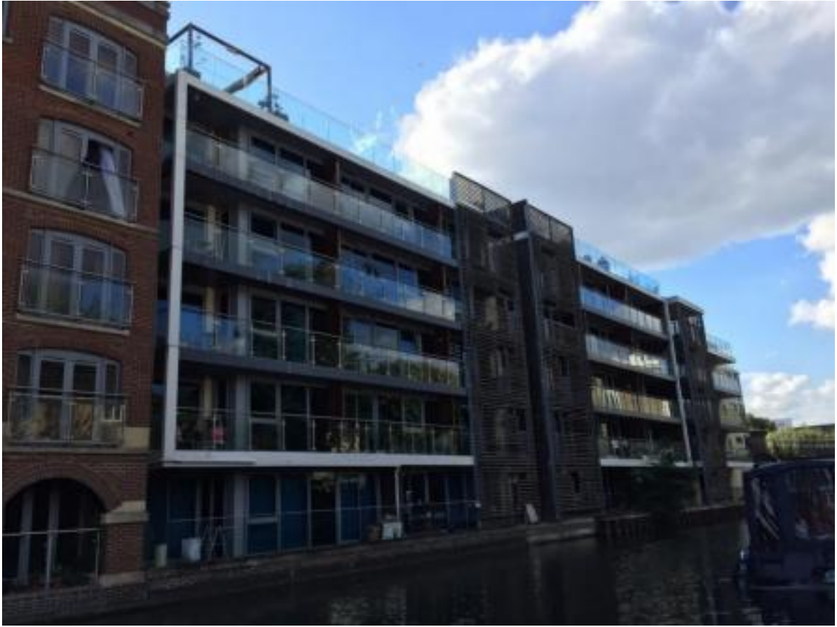
Figure 14. View of Star and Pratt Wharf from the Regent's Canal towpath.
