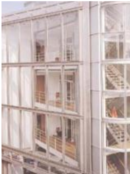
Although the floorplates are at an angle to the street, a glass outer skin maintains the building line.
