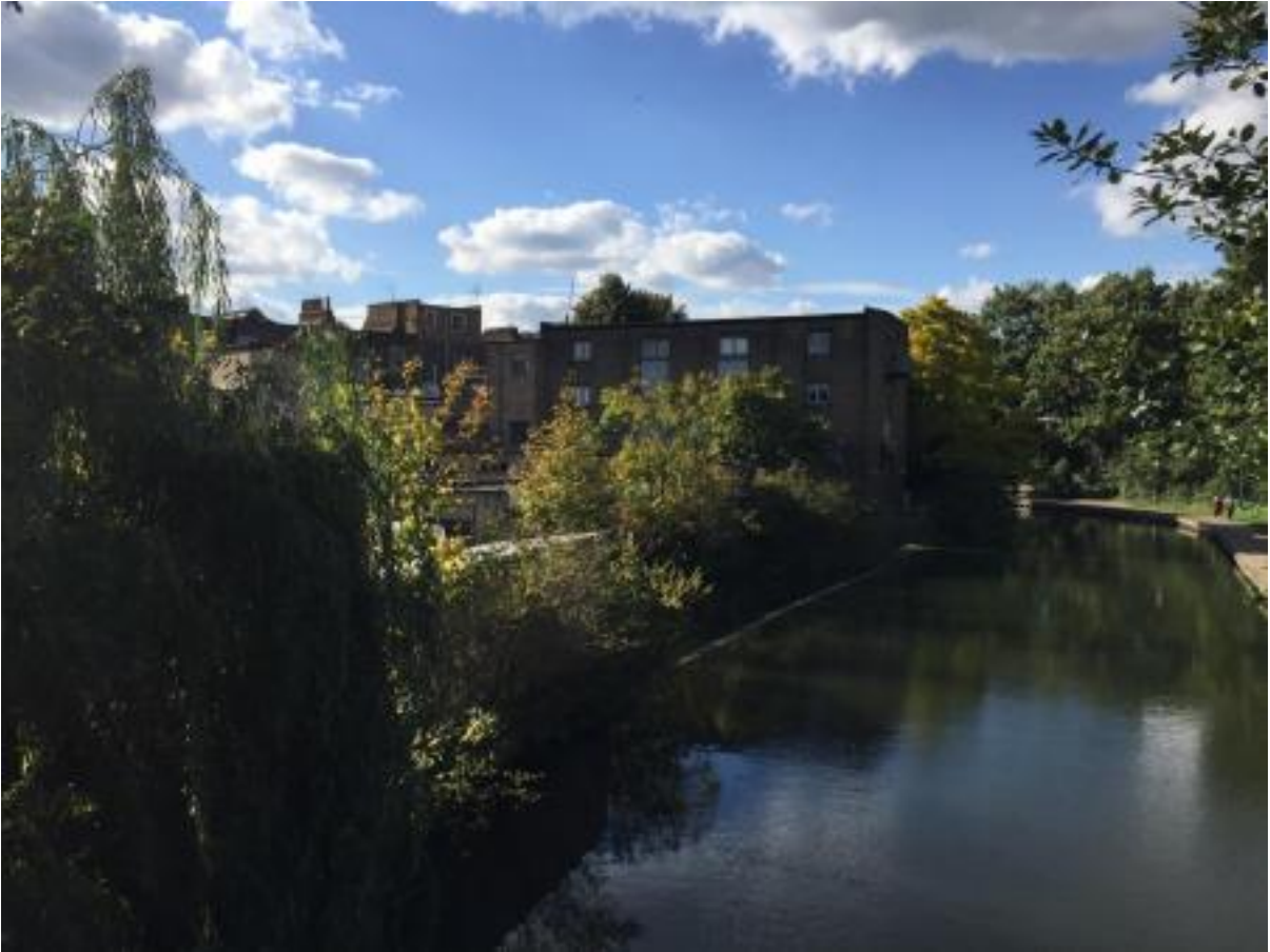
Figure 3. Appeal site viewed from Gray's Inn Bridge, with Eagle Wharf behind.
