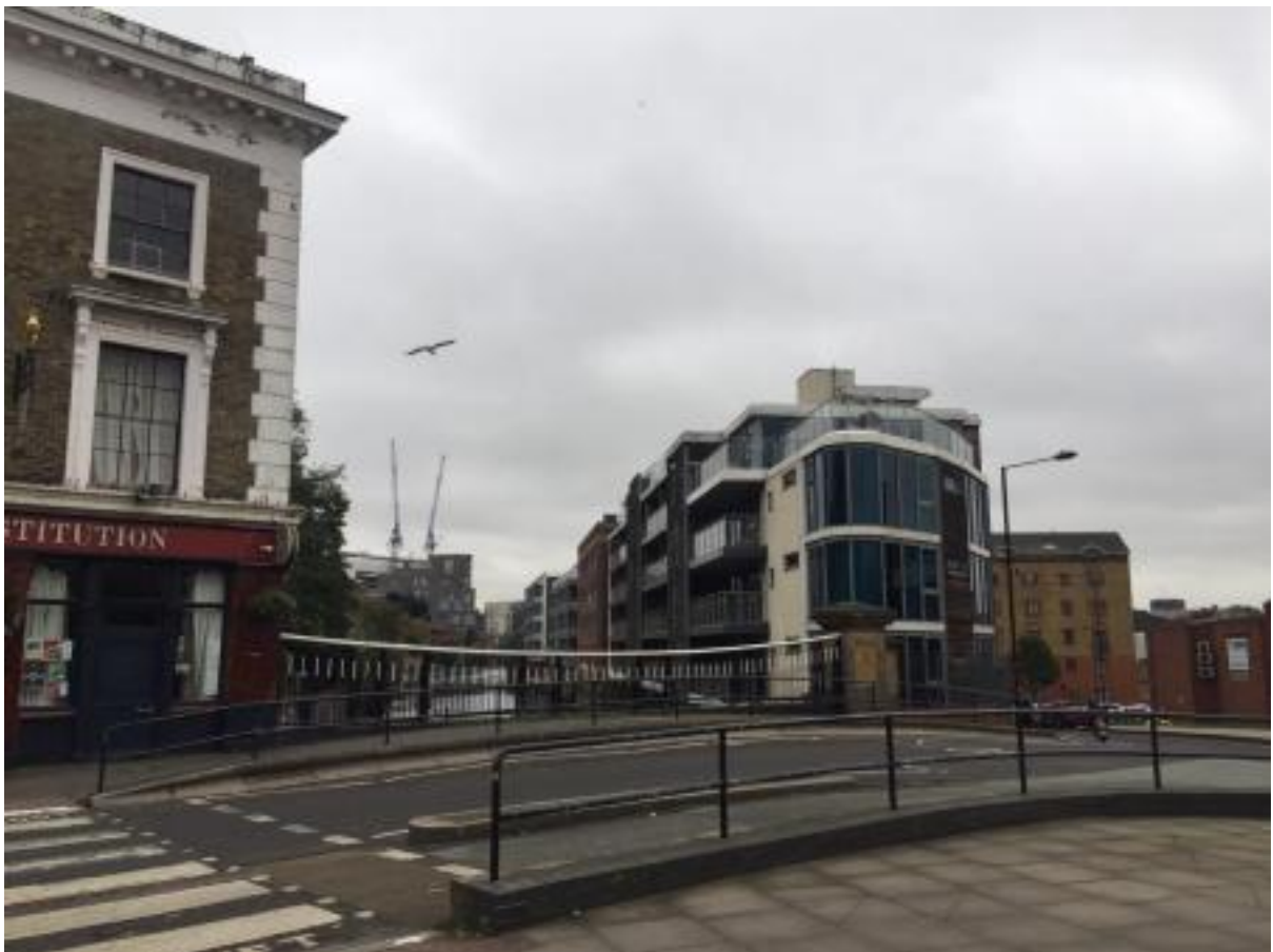
Figure 13. View of Star Wharf and Pratt Wharf viewed from Gray's Inn Bridge.
