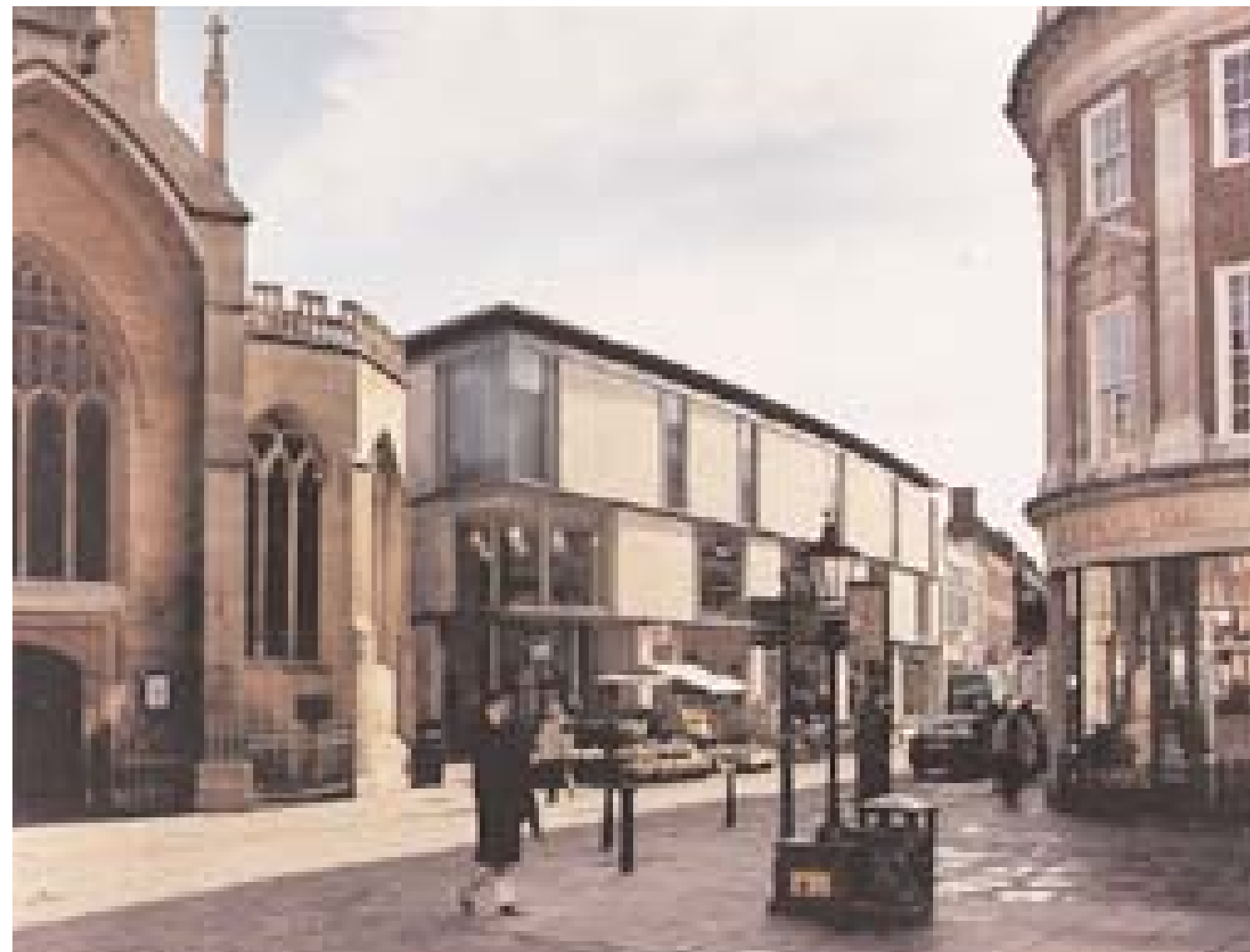
The predominantly stone elevations carry echoes of the neighbouring church.
