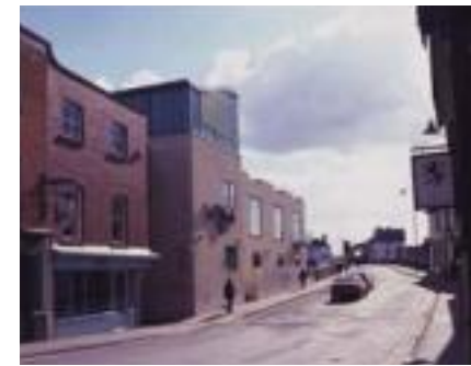
The elevation to Bridge Street is clad in bath stone.
