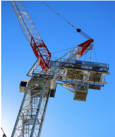
Typical Example of Luffing Tower Crane
