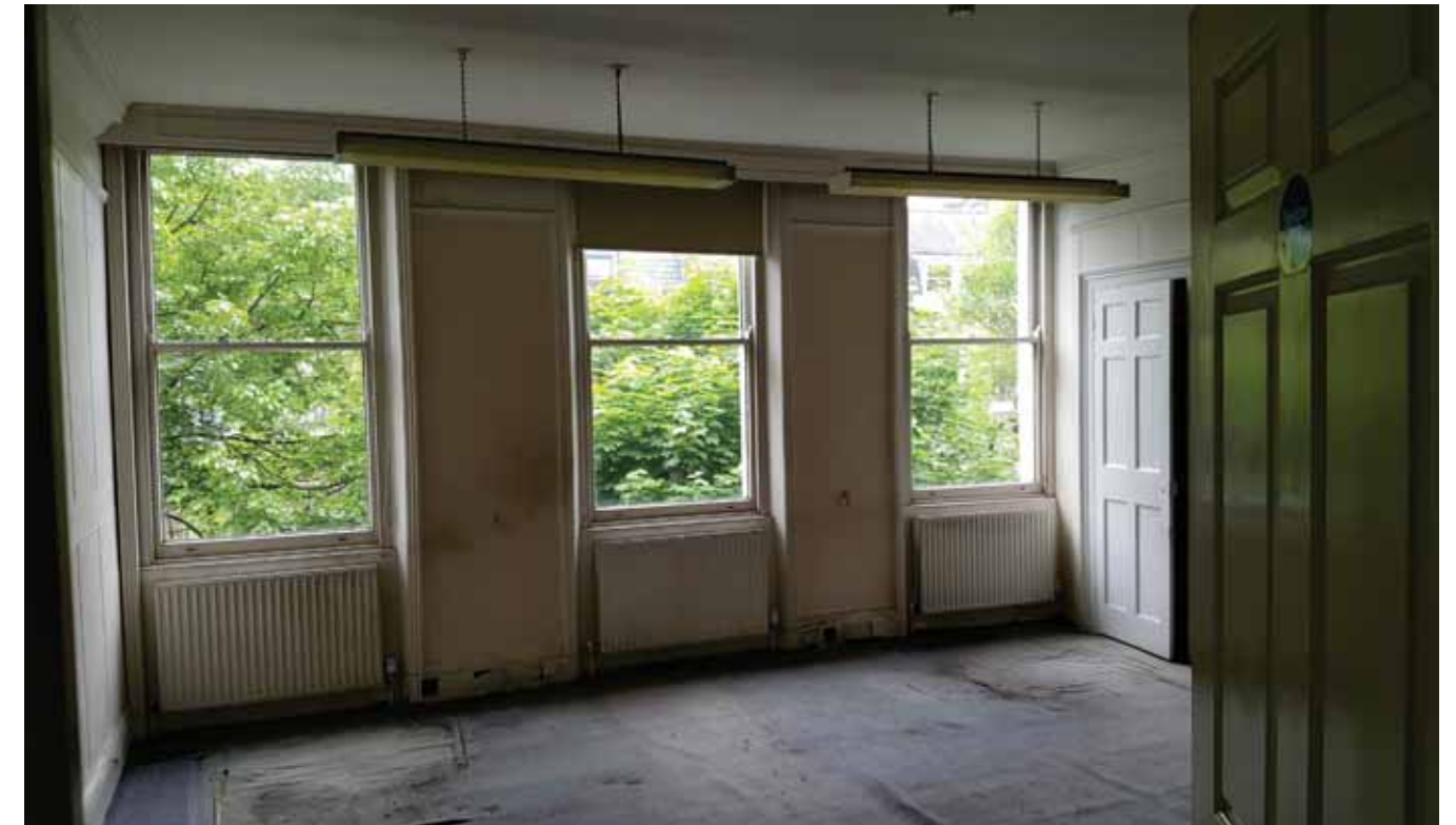
Three windows across front wall. Shutter boxes and false wall lost.
