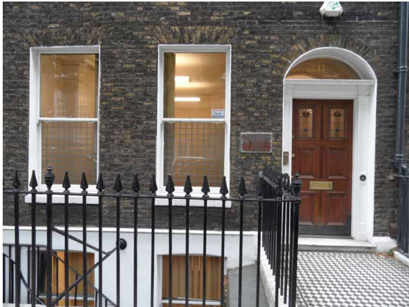
The windows at no 42 are currently all 1 over 1 pattern.
