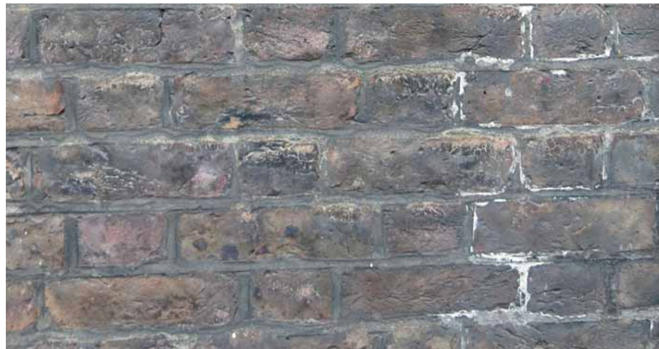
Dark multi stock brickwork with cement pointing.
