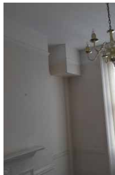
Boxing out on NE corner.
