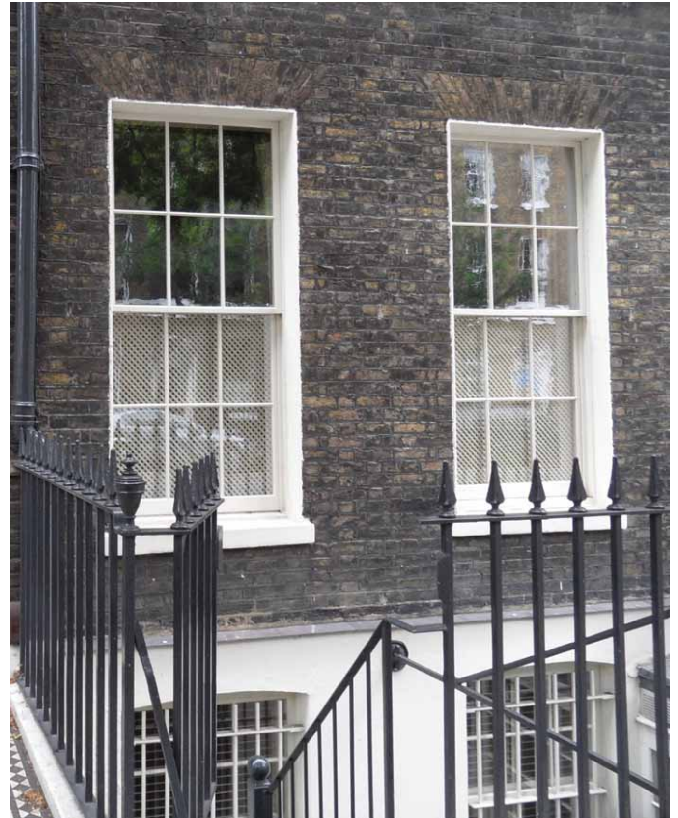
The windows at no 43 are multi pane sashes.
