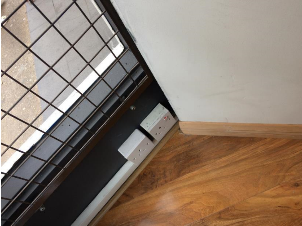
Photograph of bottom of partition and relationship with timber framed glazed shop front.
