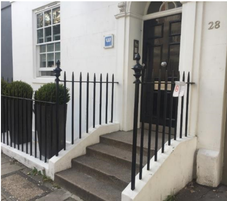
Photographs of railings with finials on 28 Percy Street, to be matched.
