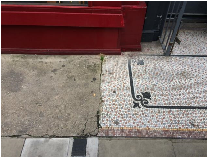
Photograph of existing mosaic and surrounding concrete finish.
