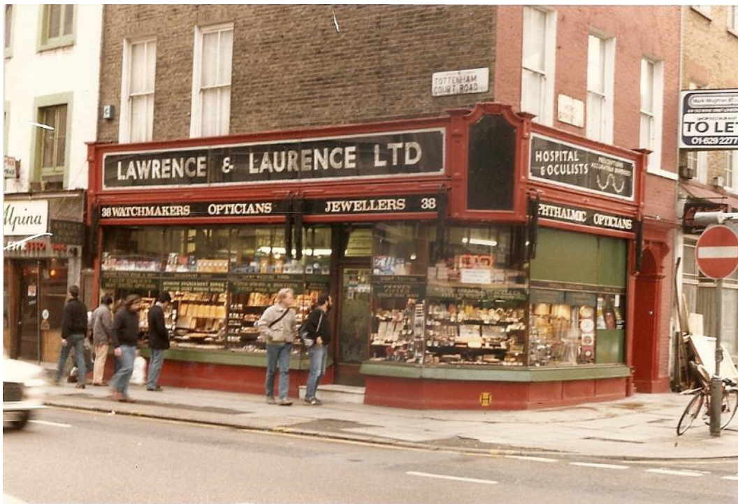
Photograph of 38 Tottenham Court Road / 20 Percy Street taken in the 1970s (prior to time of listing)
