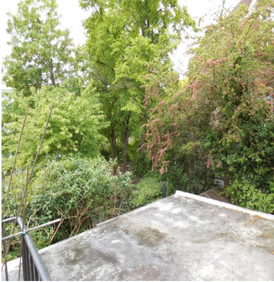
Flat roof to rear extension
