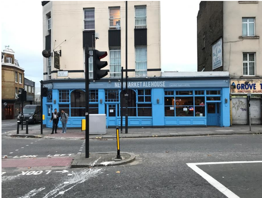
View of the site - Agar Grove Elevation (North)
