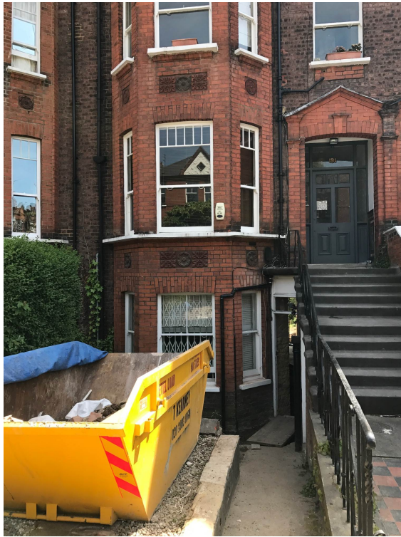
Photos of front elevation
