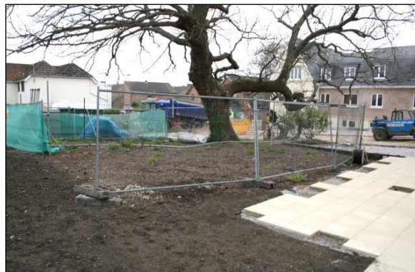
Landscaping image 2: This tree had tarmac parking within its RPA that was removed and replaced with an organic mulch near the trunk and limited no-dig surfacing on the outer edges of its RPA.
