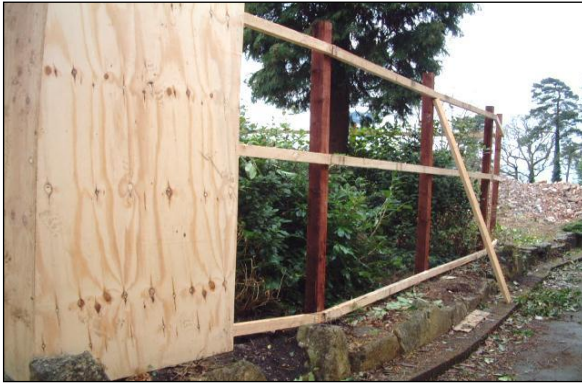
Fencing image 4: Board specification on secure wooden posts is a suitable alternative to the standard braced scaffold design.
