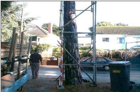
Fencing image 5: A scaffold-braced framework surrounding the trunk reduces the risk of accidental impact.
