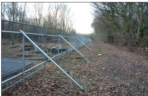
Fencing image 2: Heras fencing wired to scaffold braced posts is a robust and effective interpretation of the BS specification.
