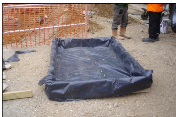
Pollution image 2: Soil bunding or a supporting framework covered in heavy-duty plastic sheeting is essential where there is a risk of spillages contaminating RPAs. This specifically applies to cement mixing areas and vehicle washing facilities.
