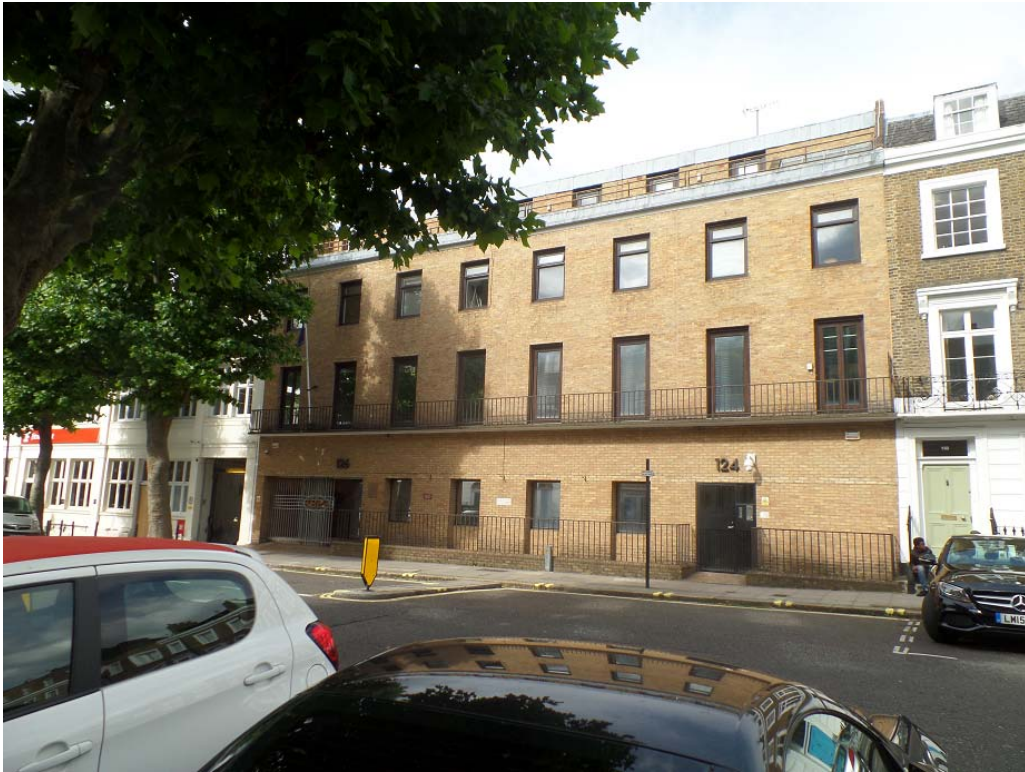
Photo 1: The existing site
