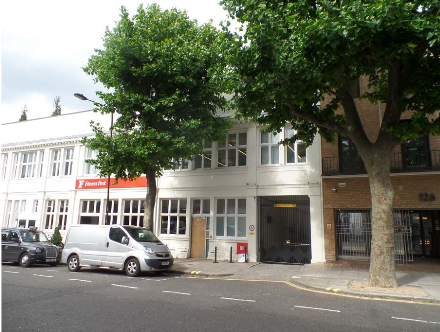
Photo 2: 128 Albert Street (front elevation)
