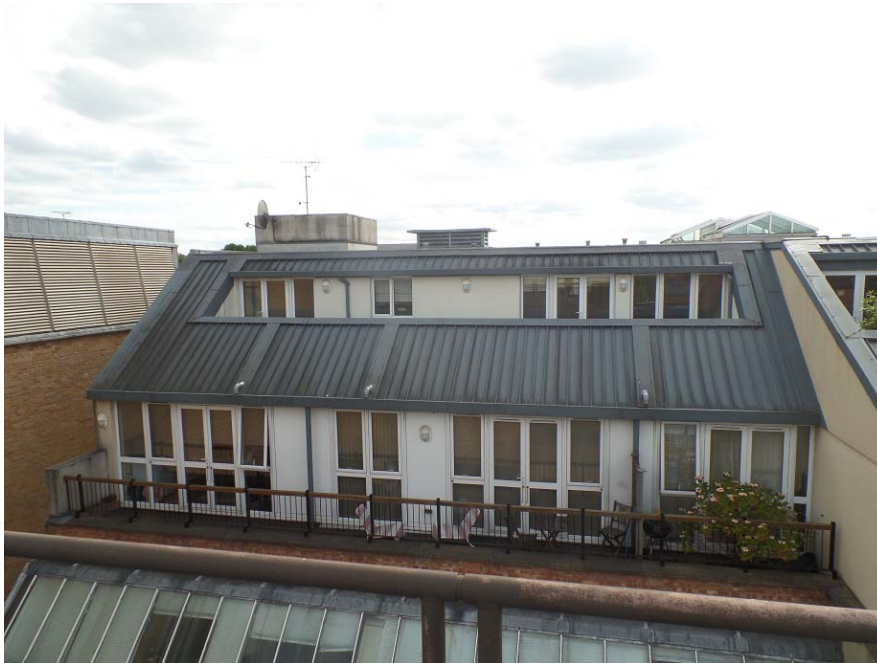
Photo 3: 128 Albert Street showing residential units (rear elevation)
