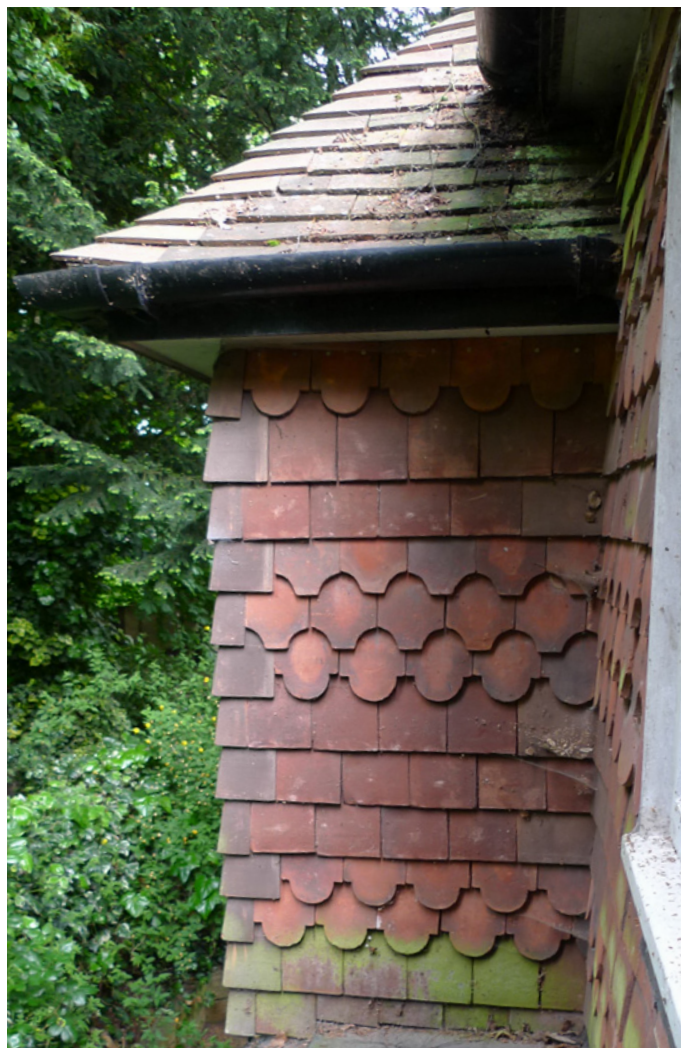
Terracotta tiles lining upper storey external walls
