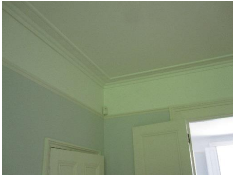
Picture rail – Painted timber picture rail. This may be a later addition.
