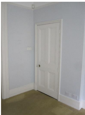
Flooring and skirting – fitted carpeted flooring over timber boarding. Taller skirting with moulded top.
