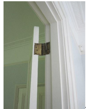
Interconnecting doors between rooms – Three panelled doors of two panels each. Typical of original construction, with wider architrave with ogee moulded profile. Doors opens into rear room with broad projecting butts.
