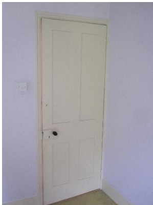
Door to room – Four panel door without panel mouldings and rim lock in moulded architrave. Probably original.
