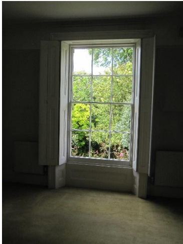
Window with shutters – Painted vertically sliding sash windows of six-over-six panes with hinged shutters fitting into shutter box with apron and soffit panels.
