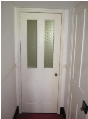
Door of lavatory – Later four panel door with upper two panels glazed with etched glass with star motif.
