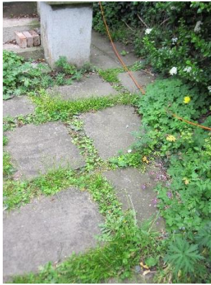
Paving near south side of house: York stone paving with wide gaps between infilled with soil. York stone possibly land on hardcore.
