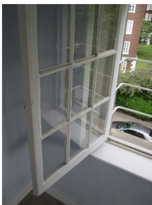
Window to rear: Hinged casement of nine panes. Thinner glazing bars suggest this is original. Window guards on the outside.
