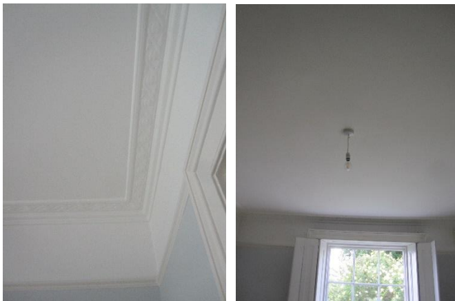
Cornice – Plaster cornice with enrichment. Overpainting suggests that it is original. No ceiling rose to this room.
