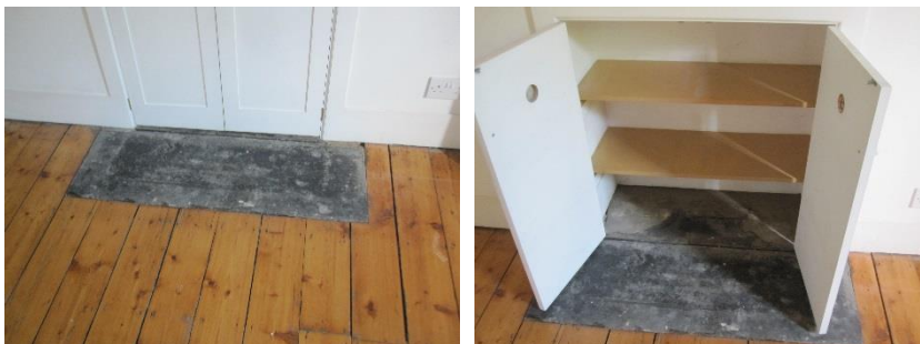
Floor and cupboard in fireplace recess: Boarded floor and hearth to fireplace (now removed) and modern cupboard inserted.
