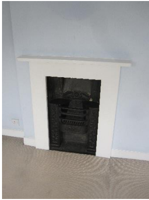
Fireplace: Painted timber surround with cast iron gate hearth covered by carpet.
