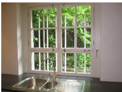
Casement and fixed light window. This is a replacement installation.
