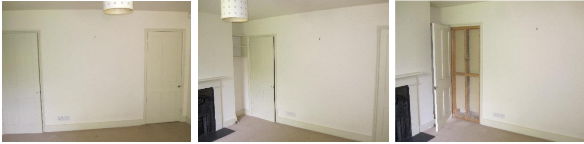
Wall to lobby to rear room – Two four panel doors with ogee moulded architecture of type. Likely to be original. Door to lobby has timber framing on the inside.
