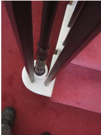
Staircase balustrade to flight to basement: Nosings to staircase over cut string – mahogany handrail, turned newel and painted sticks.
