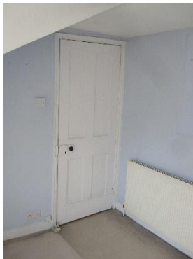
Door to room: Four panel door without panel mouldings with rim lock and architraves. Probably original.
