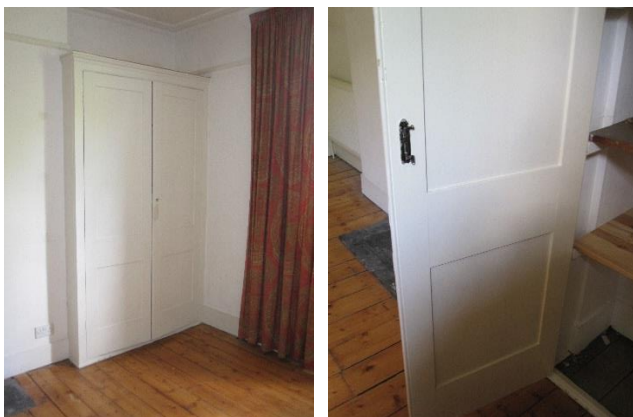
Floor and cupboard in fireplace recess: Boarded floor and hearth to fireplace (now removed) and modern cupboard inserted.
