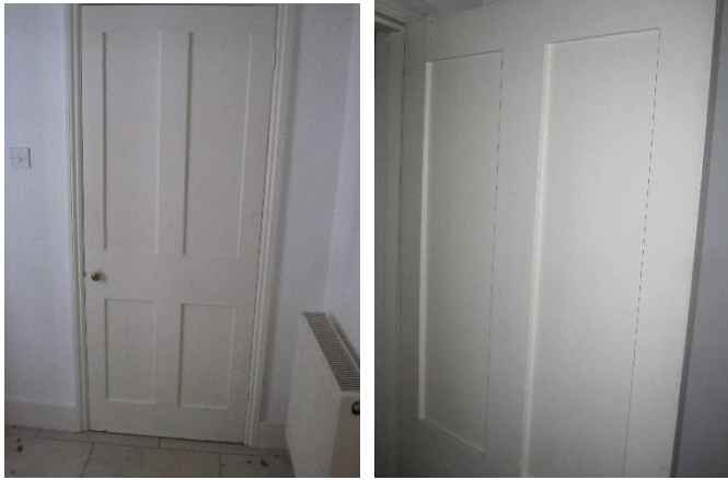
Door to space beneath front steps – Front panel door without panel mouldings of type. Likely to be original.
