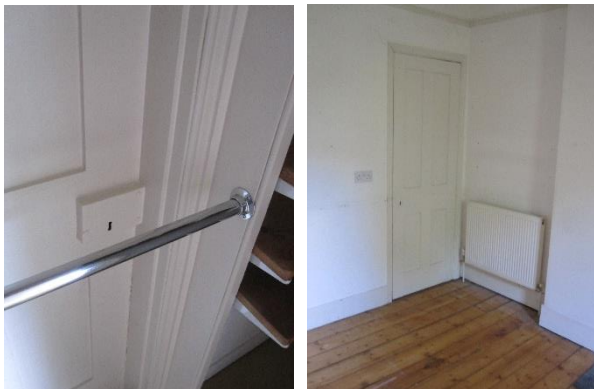
Door to cupboard: Four panel door without panel mouldings and architrave with rim lock.
