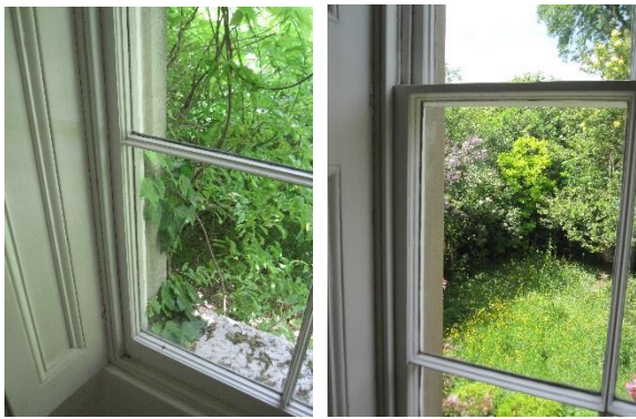
Window: Painted vertically sliding sash window of six panes over six panes with hinged shutters folding into shutter box. Glazing bars to top rail of sashes are ‘thin’ with lambs tongue mouldings but thickness of paint suggests these are replacements.
