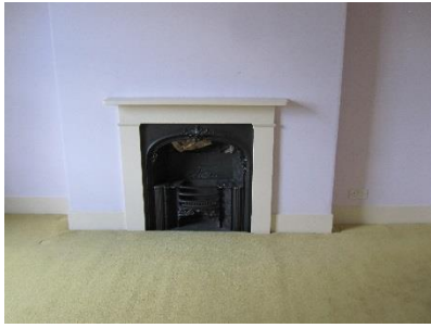
Fireplace: Painted timber chimneypiece with restrained mouldings typical of the date of construction with cast iron grate. Hearth covered by carpet.
