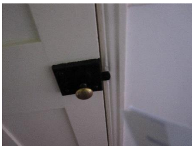
Door to cupboard at side – Four panel door with panel moulding and rim latch of original type.
