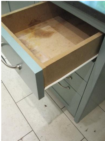
Kitchen Sink unit – Kitchen unit under window has a traditional look and has a Westmoreland slate top. The drawers have MDF carcasses so it is of recent construction, and would therefore not be considered to be part of the heritage asset.
