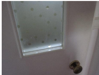
Door of lavatory – Later four panel door with upper two panels glazed with etched glass with star motif.
