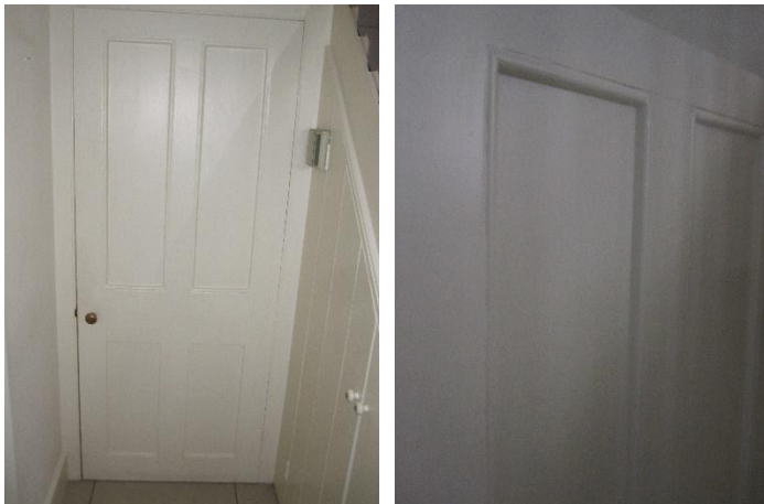
Door to back of staircase hall – Four panel door with quadrant moulding to upper two panels. This suggests that this was once glazed but now panelled in timber. Lower panel without mouldings. Glazing may have been similar to door to W.C. on the ground floor.
