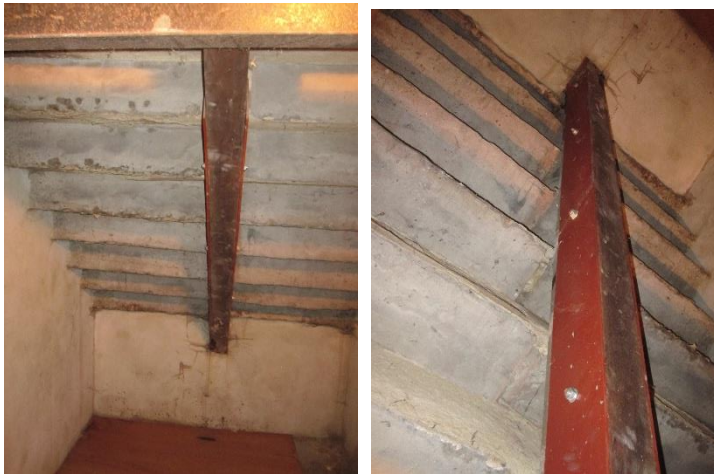
Soffit of steps to front door – stone steps supported on original timber carriage with, later steel strengthening plates, bearing on steel 'I' section beam.
