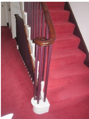
Staircase flight to first floor- Mahogany handrail with ‘Monkey Tail’ end, over turned newel and sticks laid out in a spiral.
