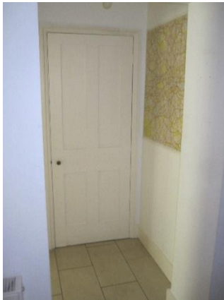
Door to hot water cylinder cupboard – Single four panel door with ogee moulded architrave. Likely to be original.
