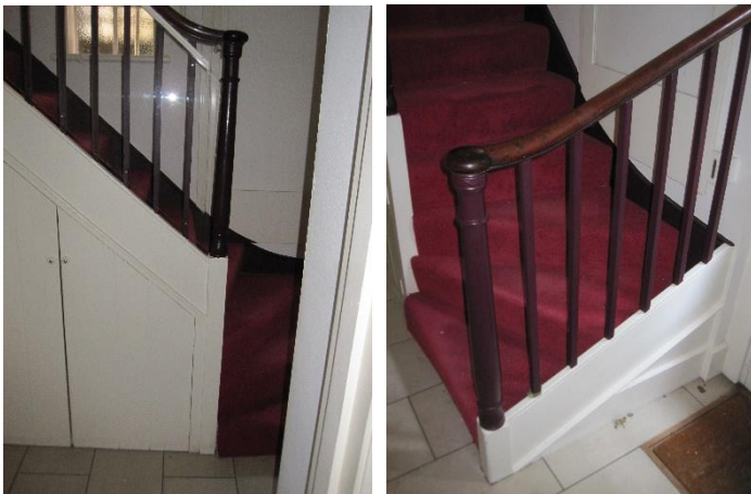
Staircase – Traditional pattern of staircase including balustrade with mahogany handrail turned newel and revel painted ‘sticks’. Cupboard beneath is 20 th Century as is the security door/panel.
