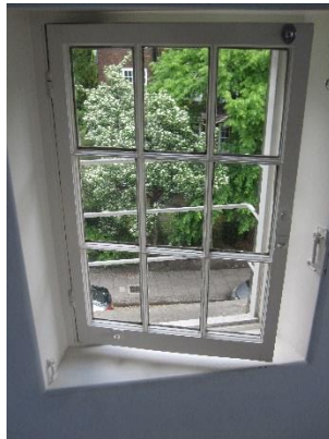
Window to rear: Hinged casement of nine panes. Thinner glazing bars suggest this is original. Window guards on the outside.
