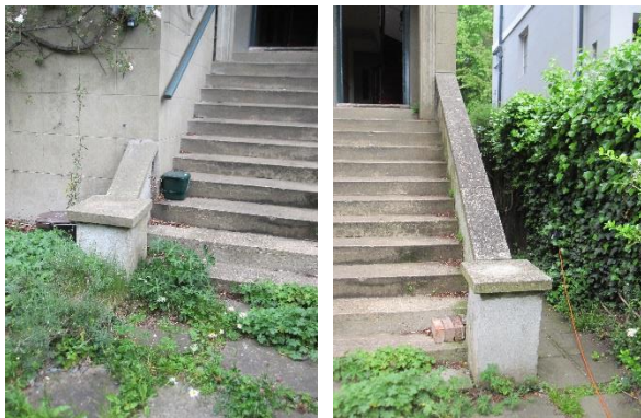
Front steps with dwarf side walls – Stone steps with cement finish. Extent of repairs to original steps unknown.
