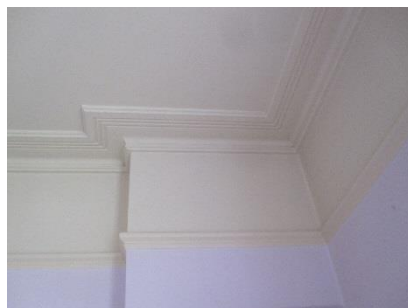
Cornice and picture rail: rim cornice but probably a replacement because not that overpainted. Picture rail maybe original.
