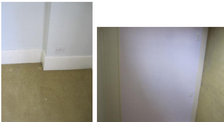
Floor: Fitted carpeted floor over timber floor boarding. Plain skirting.
