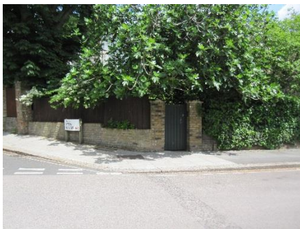
Gate to street: Late 20 th gate boarded door in between gate posts with characteristic original gate caps derived from 'Greek' architecture. Posts have either been rebuilt or certainly repointed.
