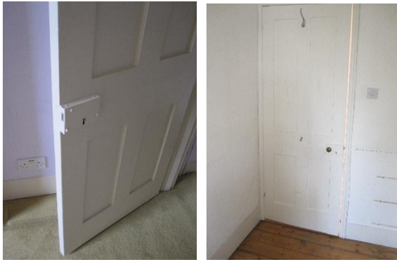
Door to room - Four panel door without panel mouldings and architrave with rim lock.
