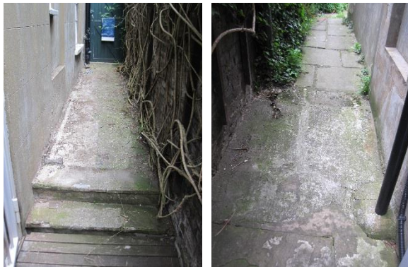
Paving side of house: Some stone with later cement repairs and lower area covered with duct boarding.
