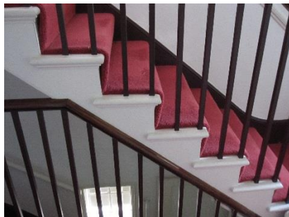
Staircase flight to first floor- Mahogany handrail with ‘Monkey Tail’ end, over turned newel and sticks laid out in a spiral.
