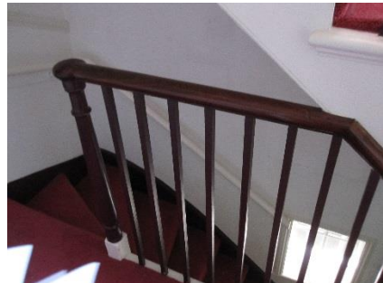
Staircase flight to first floor- Mahogany handrail with ‘Monkey Tail’ end, over turned newel and sticks laid out in a spiral.
