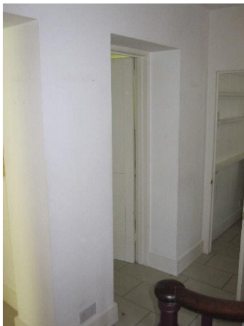
Opening to kitchen (rear room) and morning/breakfast room (front room) plaster reveals without architraves.
