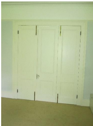
Interconnecting doors between rooms – Three panelled doors of two panels each. Typical of original construction, with wider architrave with ogee moulded profile. Doors opens into rear room with broad projecting butts.
