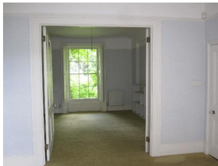
Interconnecting doors between rooms – Three panelled doors of two panels each. Typical of original construction, with wider architrave with ogee moulded profile. Doors opens into rear room with broad projecting butts.
