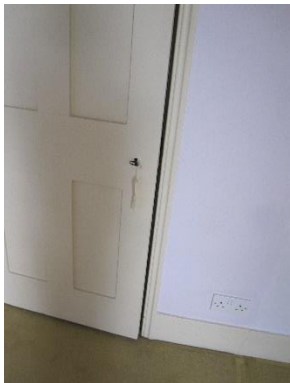
Door to cupboard – Four panel door without panel mouldings and architrave with rim lock.
