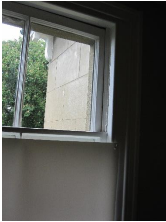
Window – Vertically sliding sash windows of three-over-six panes.
