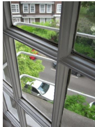
Window to rear: Hinged casement of nine panes. Thinner glazing bars suggest this is original. Window guards on the outside.
