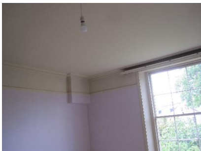
Cornice and picture rail: rim cornice but probably a replacement because not that overpainted. Picture rail maybe original.
