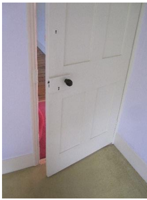
Door – Four panel door without panel mouldings architrave. Probably original.
