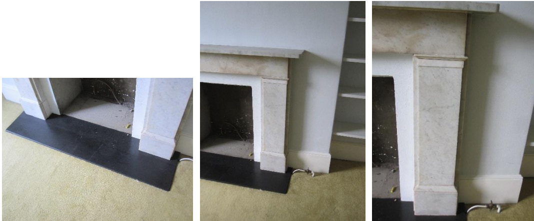
Fireplace – White marble chimney piece with restrained mouldings typical of the date of construction without grate and with later slate hearth. Original hearth likely to be beneath.
