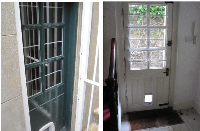
Door to outside – Modern half glazed timber door with cat flap and security bars.
