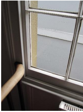
Staircase window – Vertically sliding sash window and apron panel beneath. Probably original.
