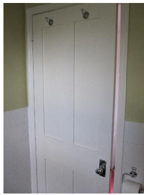
Door – Four panel door without panel mouldings architrave. Probably original.
