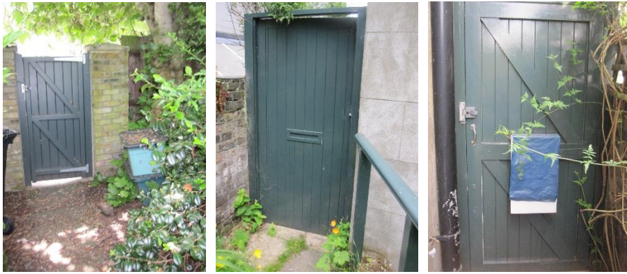
Rear and side gates – Painted timber boarded door with frame and ledges. Letterbox to side gate.
