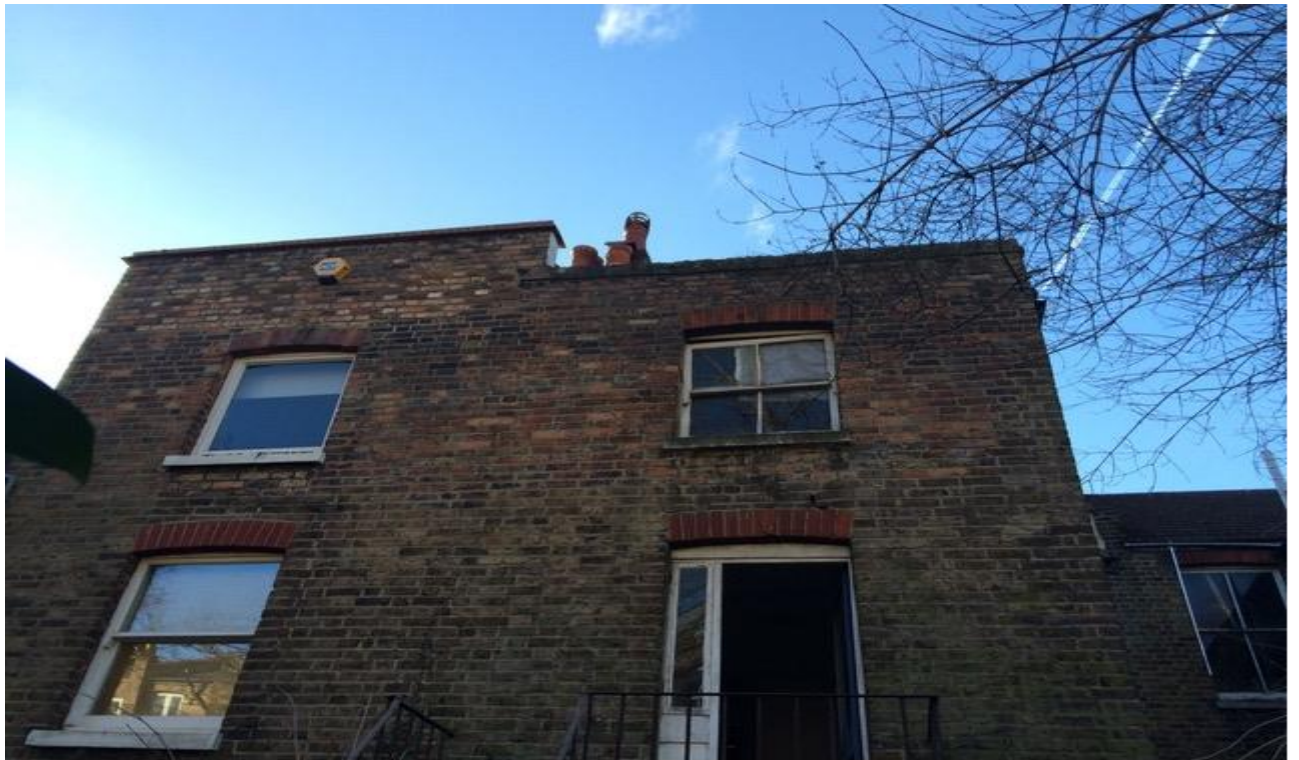
Photograph 7. Rear roof parapet
