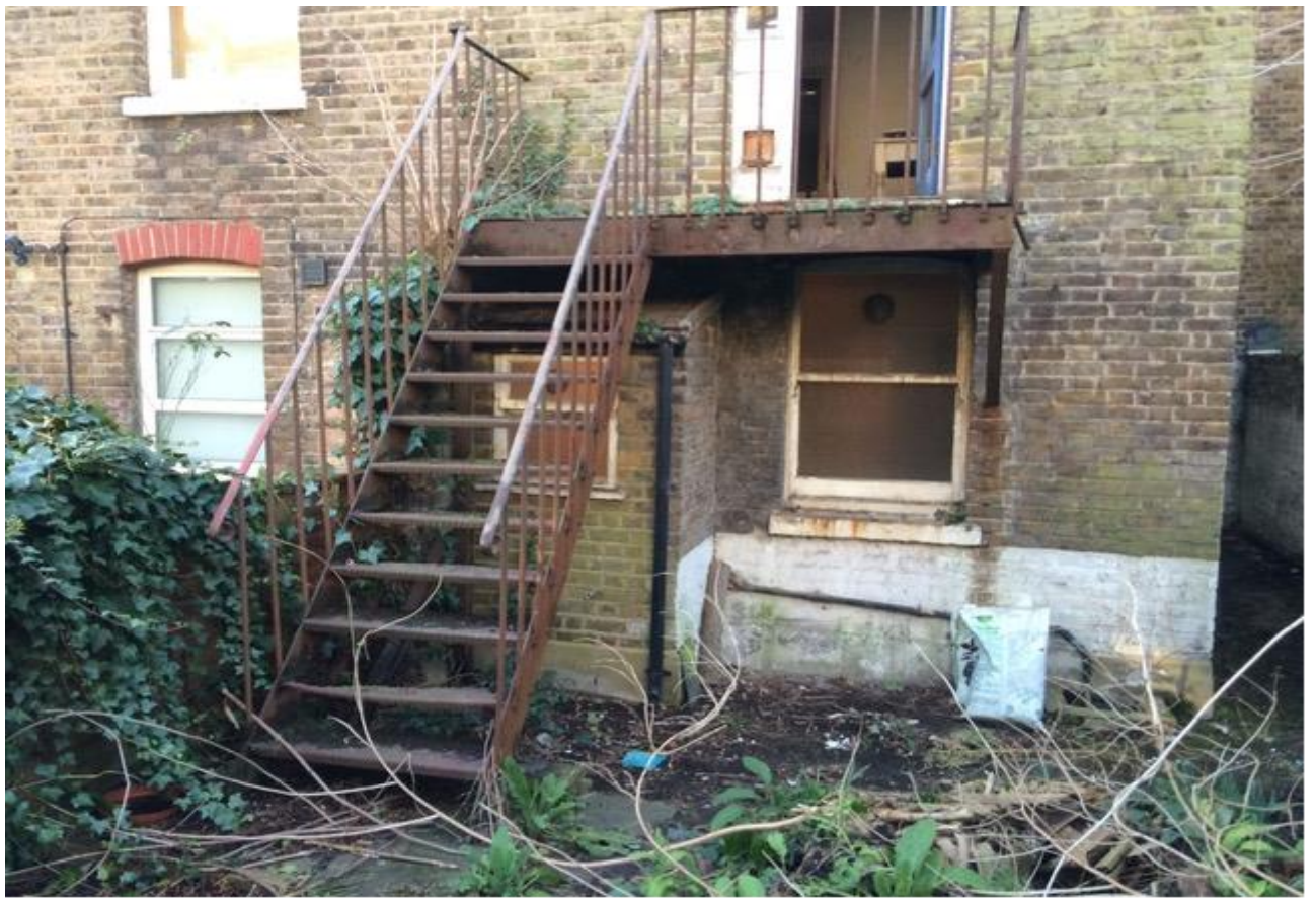
Photograph 5. Rear existing stairs
