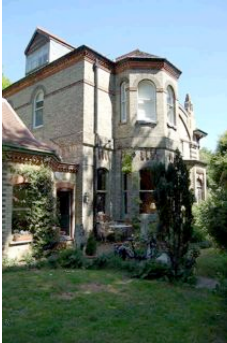
VIEW OF THE TWO STOREY ADDITION ADDED TO THE ORIGINAL VILLA – THE LOGS – ADDED CIRCA 1950's TO CREATE THE HOUSE NOW KNOWN AS 20 WELL ROAD. THE FURTHER ADDITION OF THE SINGLE- STOREY OCTAGONAL SIDE EXTENSION ADDED 1987 CAN JUST BE SEEN ON THIS PHOTOGRAPH
