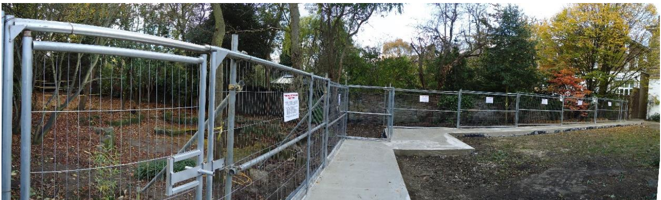
Figure 5. Photograph to illustrate installed protective fencing
