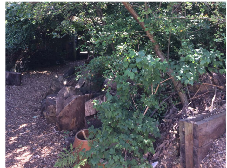
⑥ view of existing mound and loose timber edge to be removed
