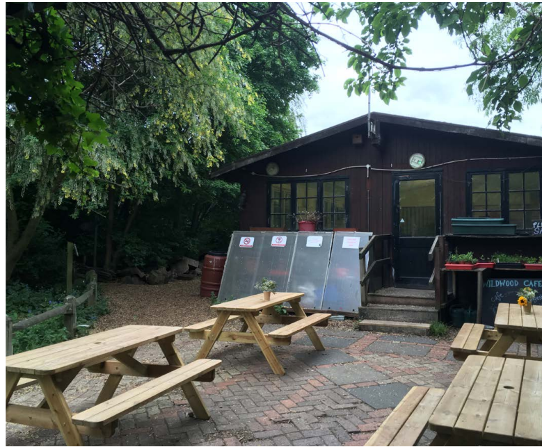
① view of Southern edge of existing building and brick paver to be demolished (learning space)
