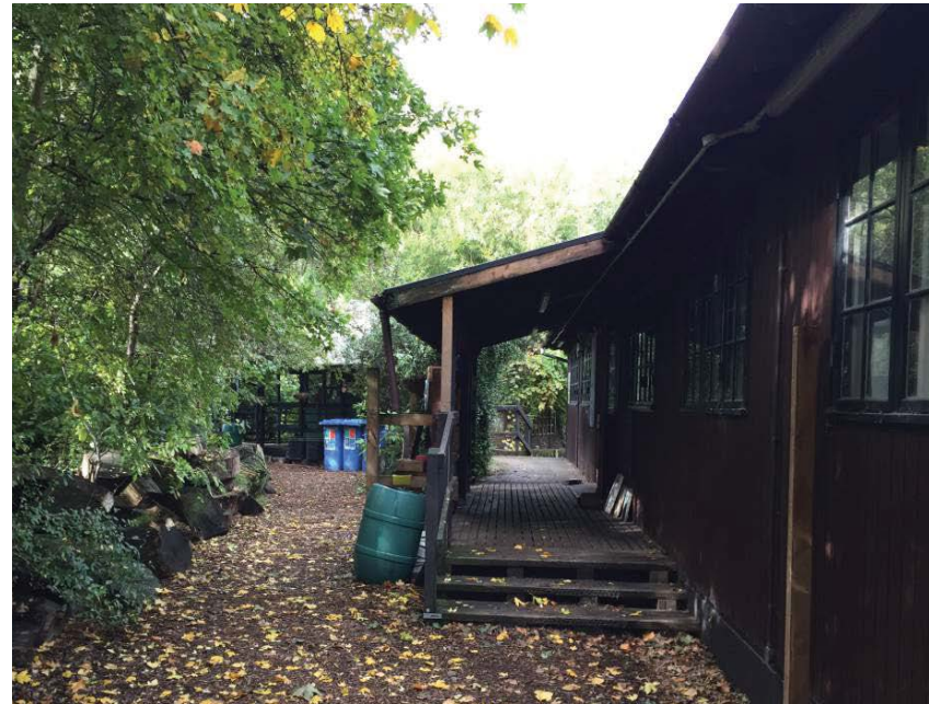
② view of external wooden deck and canopy to be demolished
