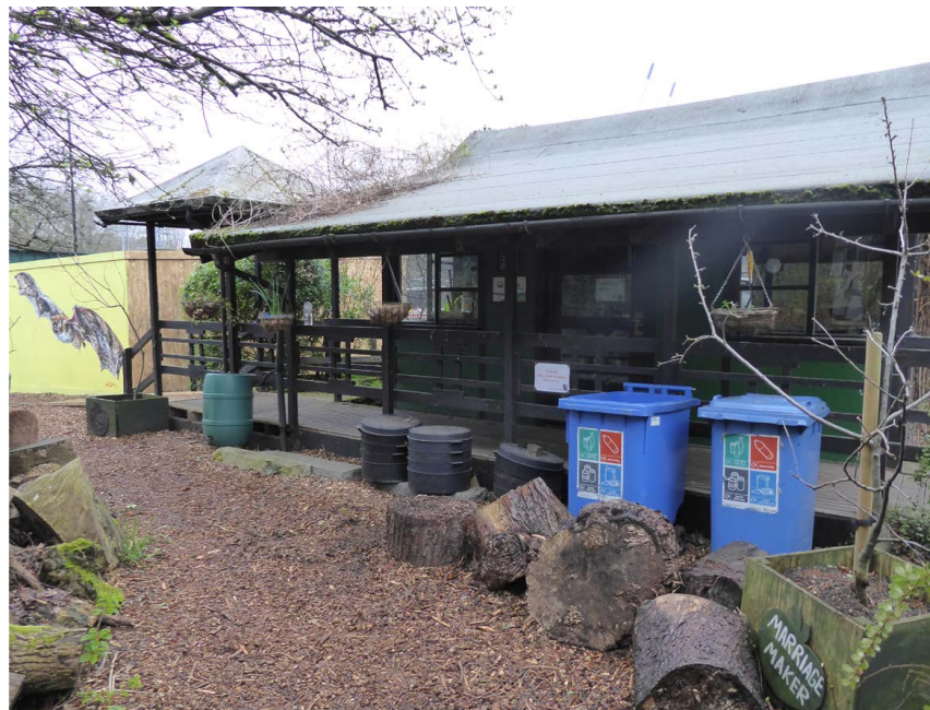
④ view of Western edge of existing building to be demolished
