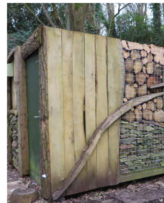
Example of storage container, clad to minimise visual impact
