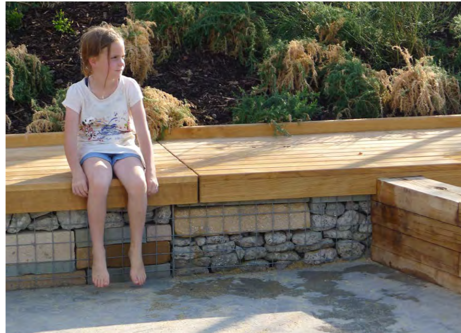
Example of gabion seating with timber surface - at Camley Street charred larch is proposed to match the new building
