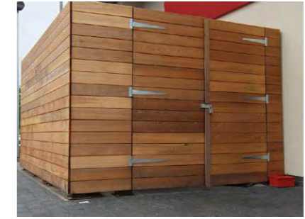
Example of timber, lockable bin store with open roof
