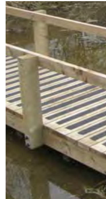
There will be timber decking to the canal and narrow boat as a break-out area from the visitor centre. The pond dipping platform will be repaired and re-surfaced with new anti-slip timber decking
