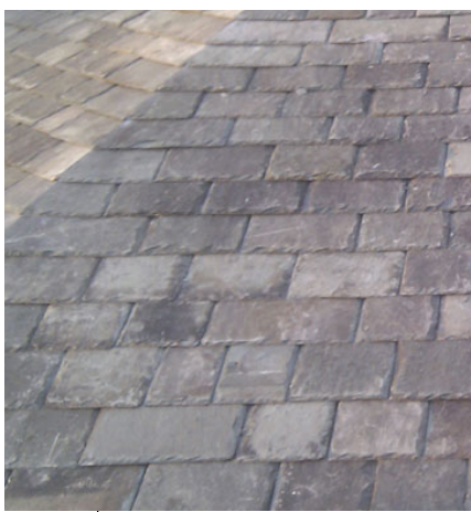
Natural slate roof mitered corner
