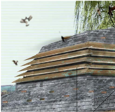
Copper cladding for fins at roof chimney
