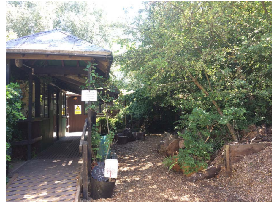
③ view of ramp, handrail, side wall of volunteer room and canopy to be demolished
