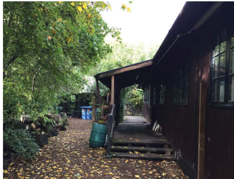
② view of external wooden deck and canopy to be demolished
