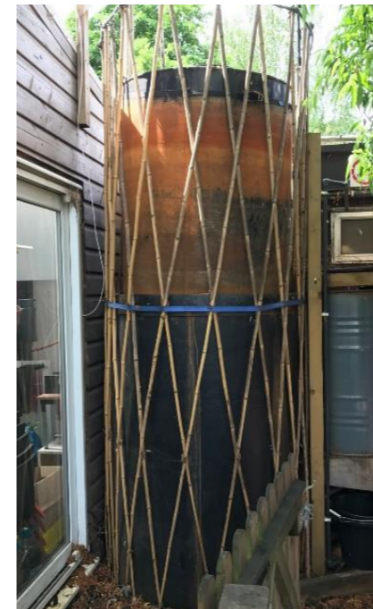
⑨ anaerobic digester system to be removed to be reused at another site (biogas storage tank)
