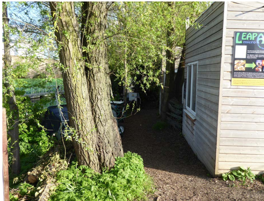
⑦ view of corner of existing building containing anaerobic digester to be demolished and existing willow tree to be removed
