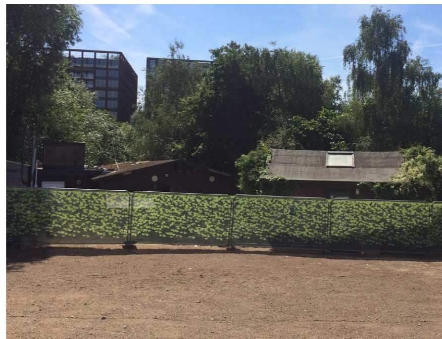
⑤ view of North edge of existing building to be demolished
