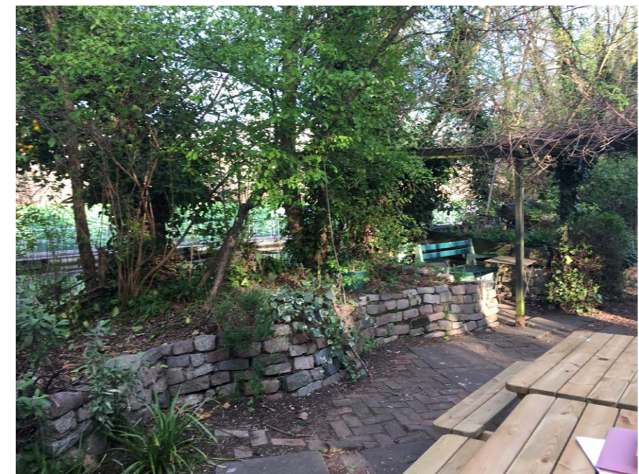
⑭ existing raised flowerbed to be retained, brick paving to be removed
