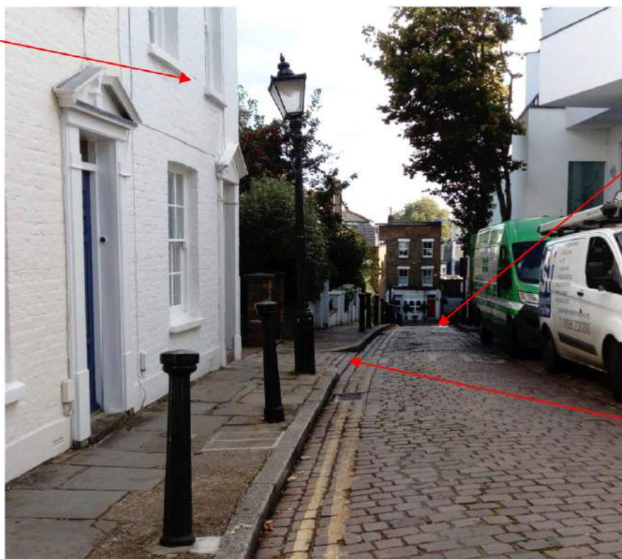
Photo 3: Carriageway of Back Lane, looking south-east. The footway slopes away from No.5, and the carriageway slopes to the south-east. Also visible is the slight drop between the Back Lane footway and the access passageway to No.5a.
