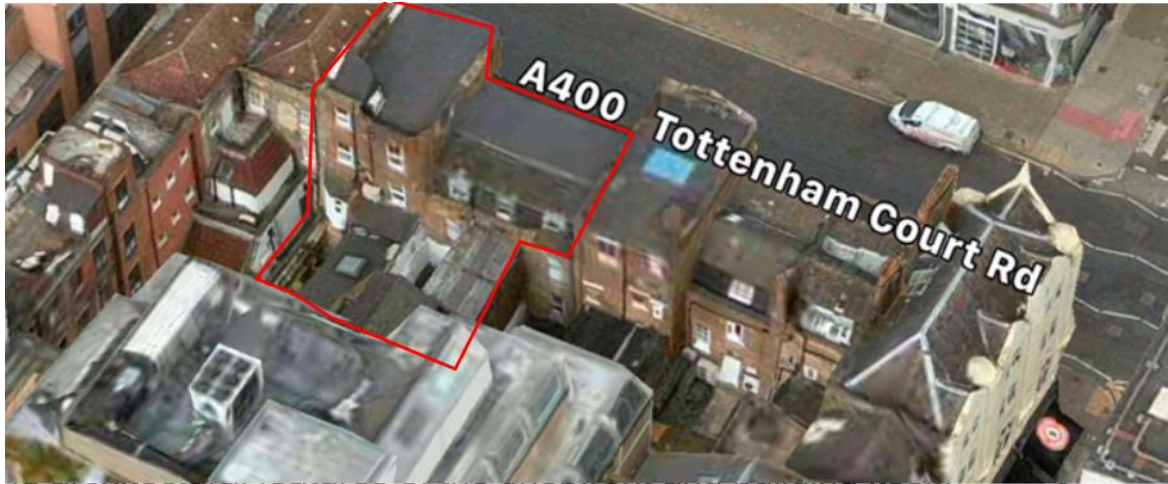
Figure 1. The rear/back of the appeal site terrace which shows a consistent and clear pattern of low scale rear extensions except where the end properties form a junction plot with neighbouring street.
