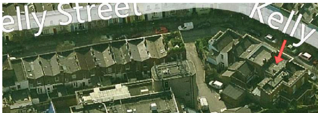
Rear of Kelly Street.
