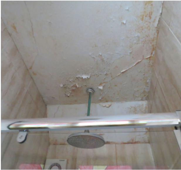
fig 6 & 7. 98 Highgate West Hill - internal and external damp
