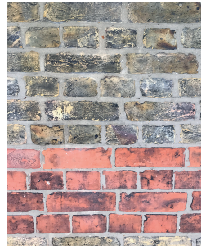
Cleaned Brickwork
