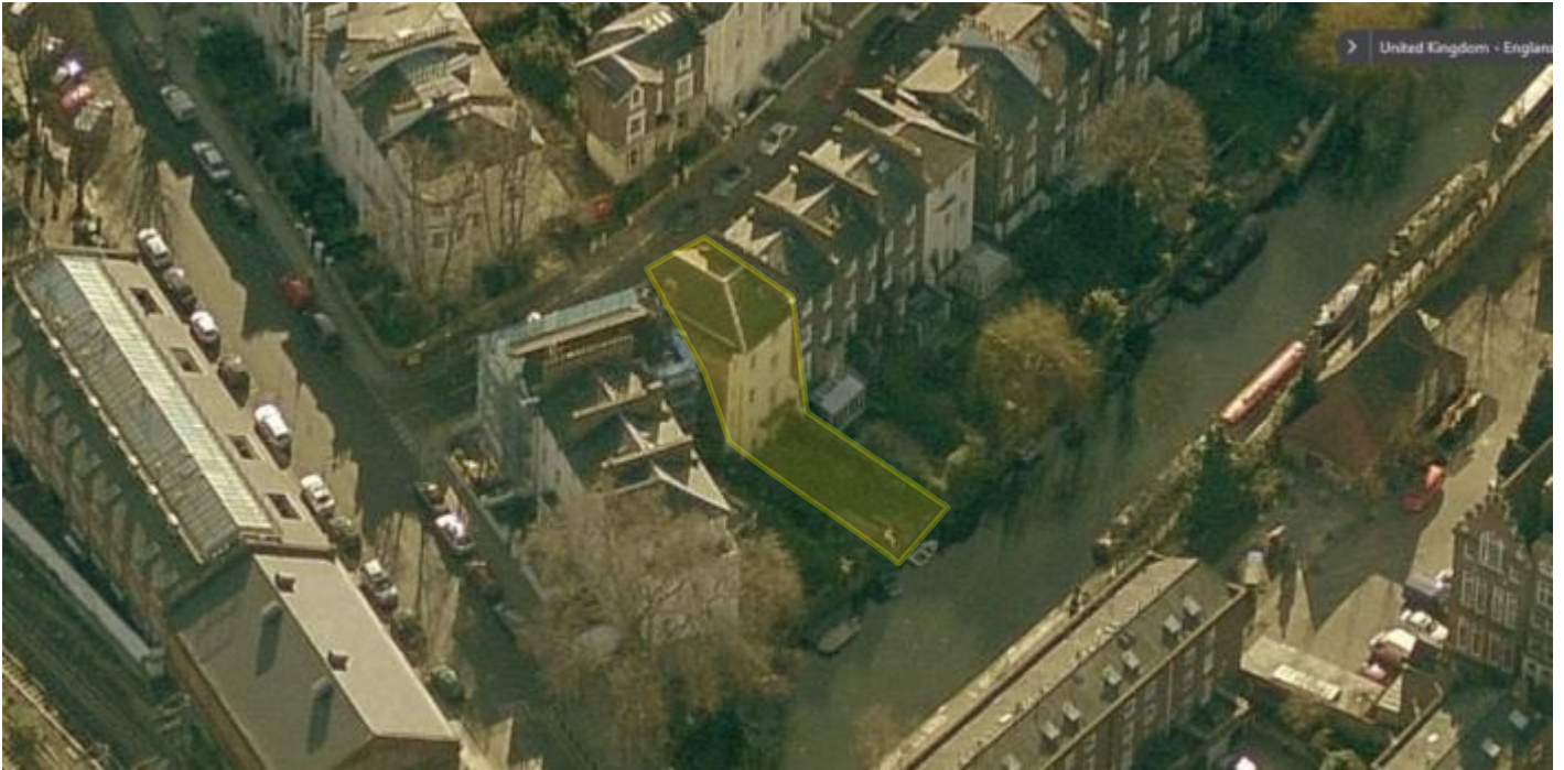
(1) Aerial photo 1 (from the North)
