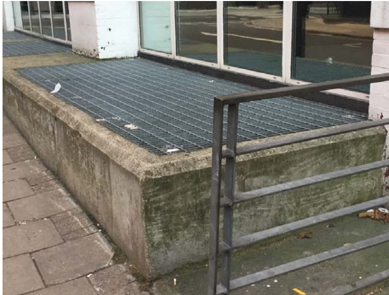
Photograph of Existing Metal Grilles to Top of Lightwell
