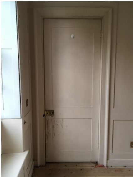
EXISTING DOOR D300 REHUNG TO OPEN WIDER THAN 90°
