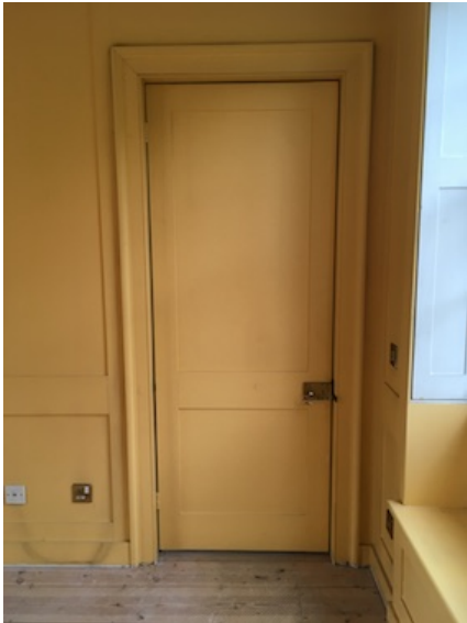
EXISTING DOOR D302 REHUNG TO OPEN WIDER THAN 90°
