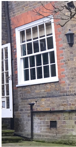
WINDOW TO BE REPLACED BY DOOR D118
