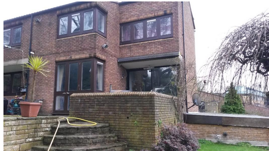
Right: View of rear of property (north west elevation) with swimming pool at lower ground floor level on right
