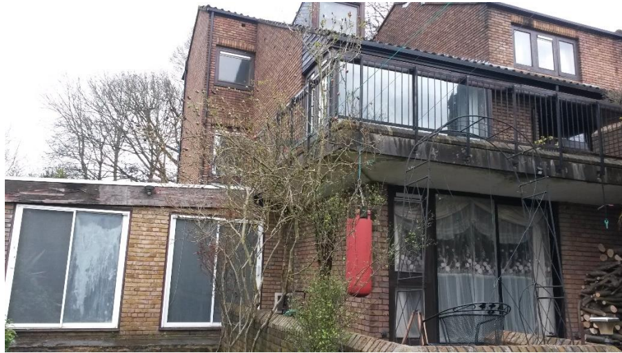
Left: View of front of property (south east elevation) from front garden at lower ground floor level.
