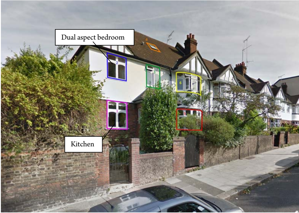
Photograph 3: Front elevation of 1 and 1A Chetwynd Villas (ignore numbering)
