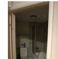
Basement front bathroom
