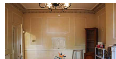
Ground floor front room spine wall
