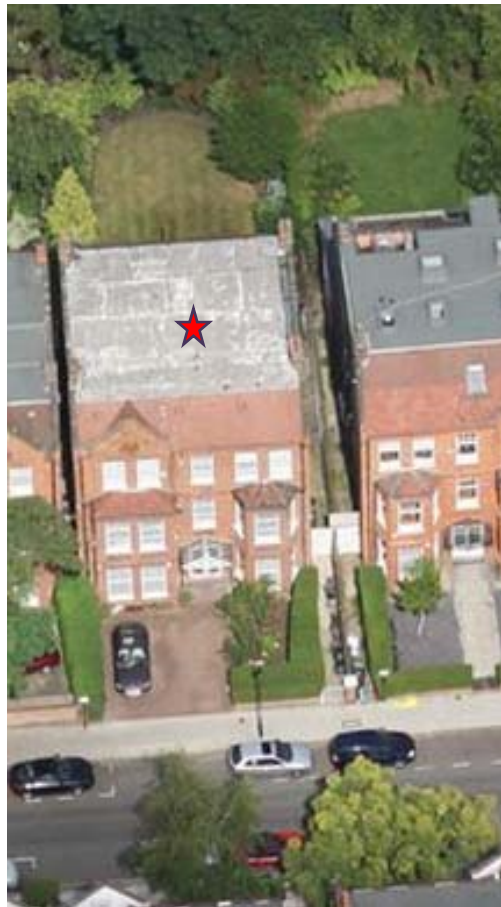
Figure 2: Birdseye View from south
