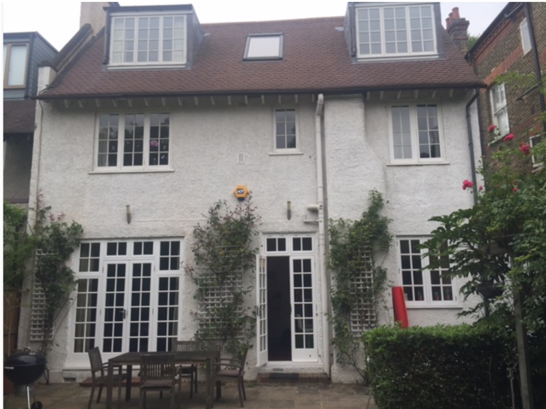
Photo 4: Existing rear elevation
