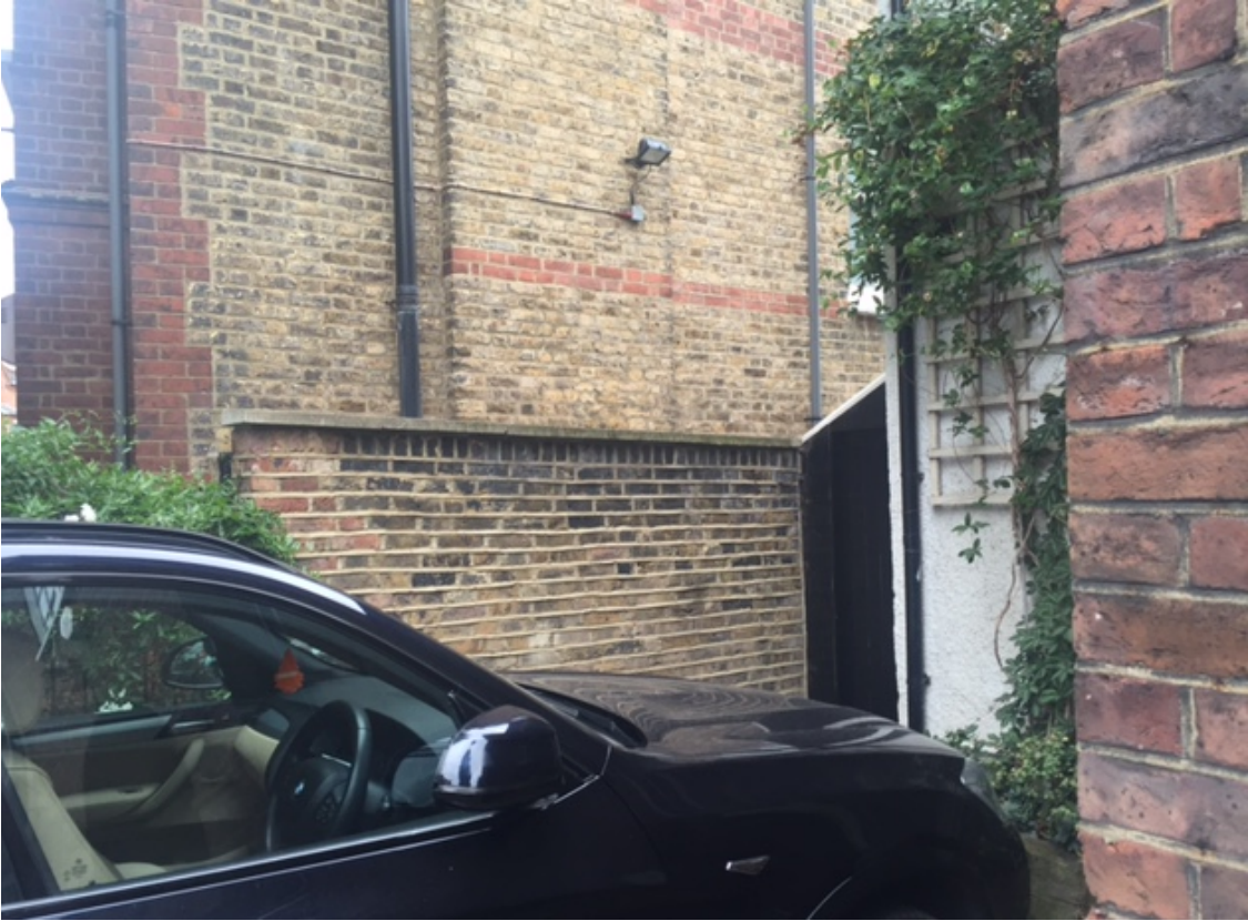
Photo 3: Showing the existing higher section of wall that will be matched
