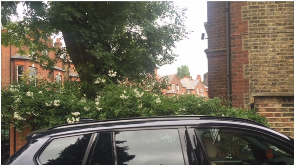
Photo 2: Section of wall to be raised
