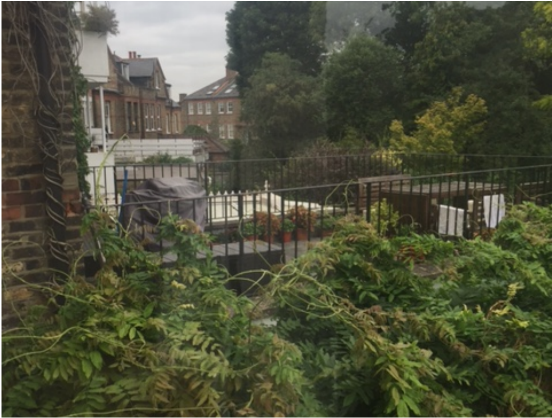
Photo 5: Rear extension at no.12
