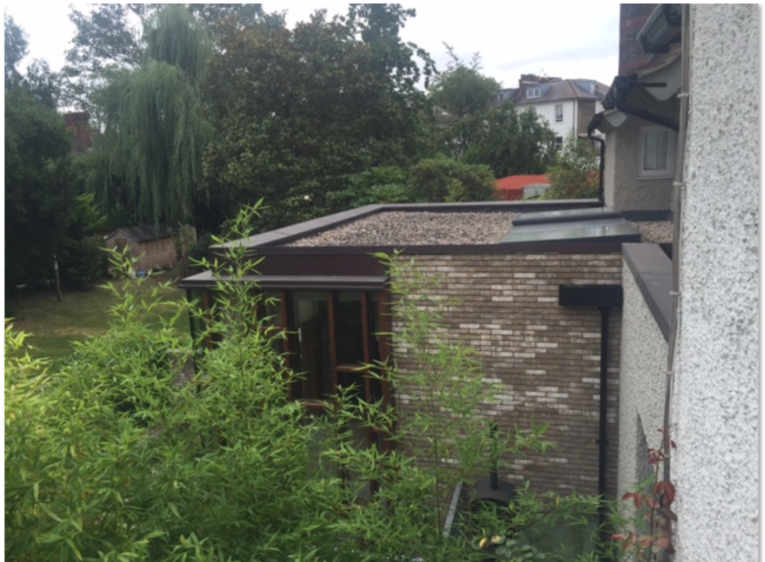
Photo 6: Rear extension at no.8
