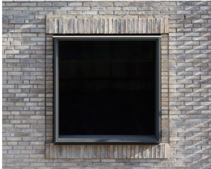
Turned brick & window cuff detailing
