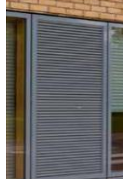
C. LOUVRES GLAZED INTO CURTAIN WALL
