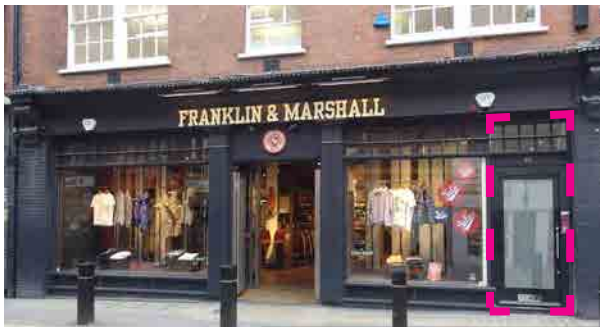
Existing Shopfront 47-49 Neal Street
