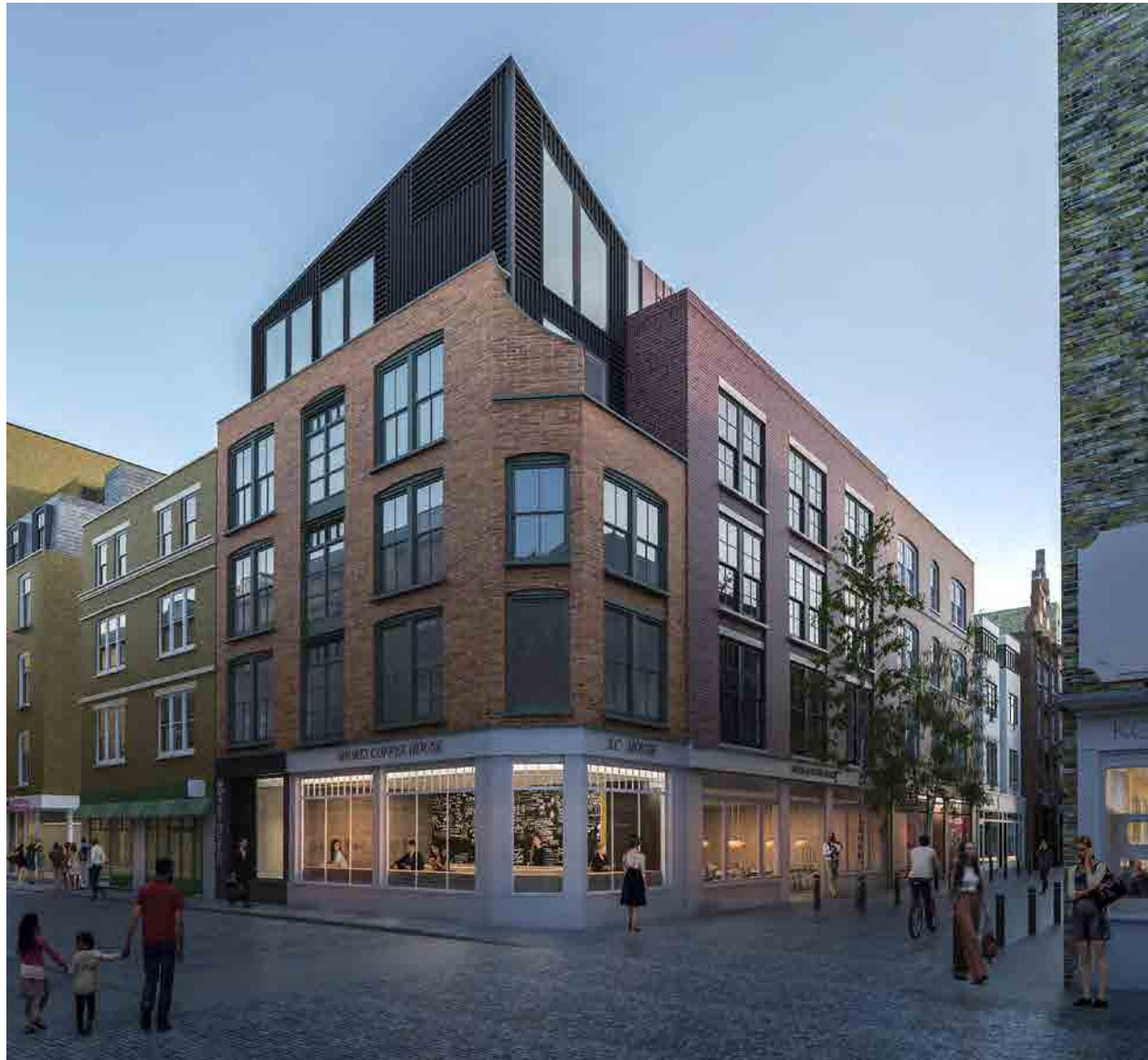
Proposal viewed from the corner junction between Neal Street and Shorts Gardens
