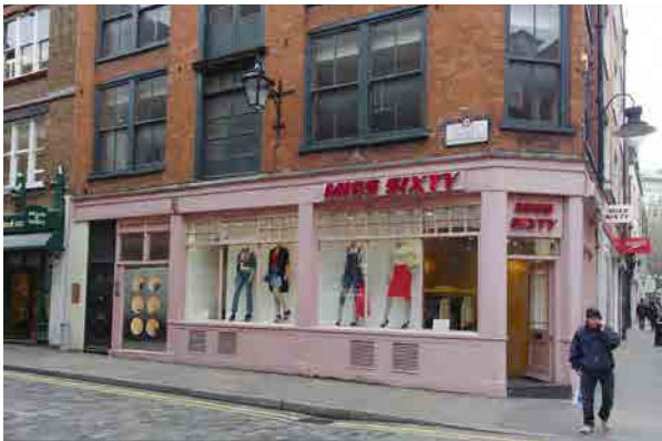
Existing shop front 39 Neal Street
