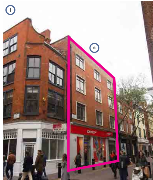
Replace poor 1950s facade
