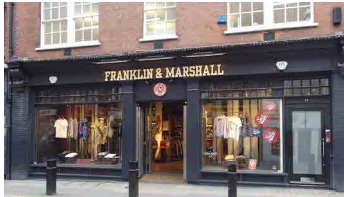
Shopfront and office entrance (47-49 Neal Street)
