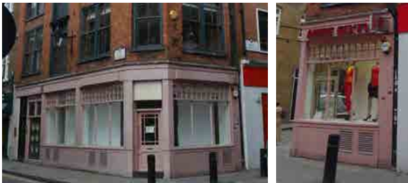
Existing shop front 39 Neal Street
