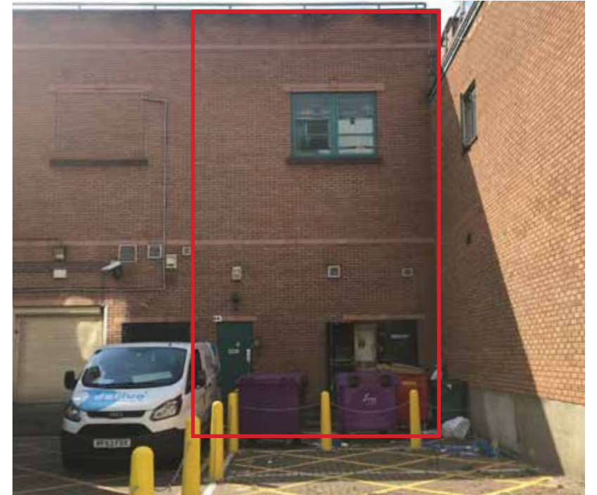
Existing Rear View
