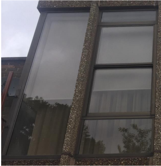
Photograph of existing tinted bay windows.
