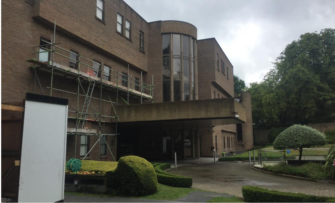
Photograph of existing entrance to Mount Tyndal
