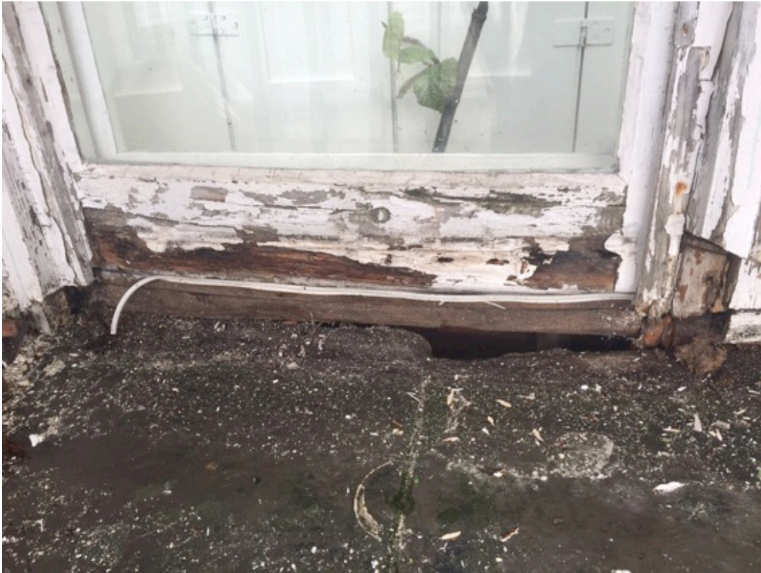
Photograph 5 – Gap between the balcony and main building indication it was not a cantilever design.
