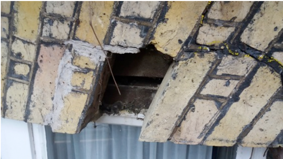
Photograph 6 – Curved steel support below the balcony.
