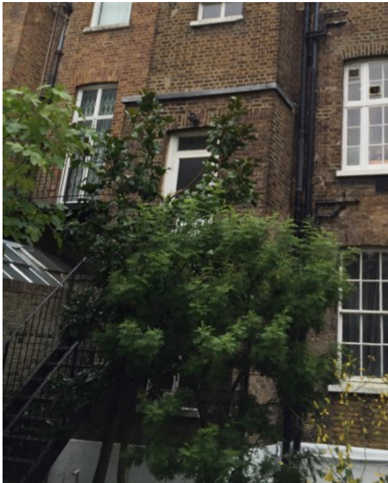
Photograph 4 – Full metal balcony and railings to rear facade (LHS of picture)
