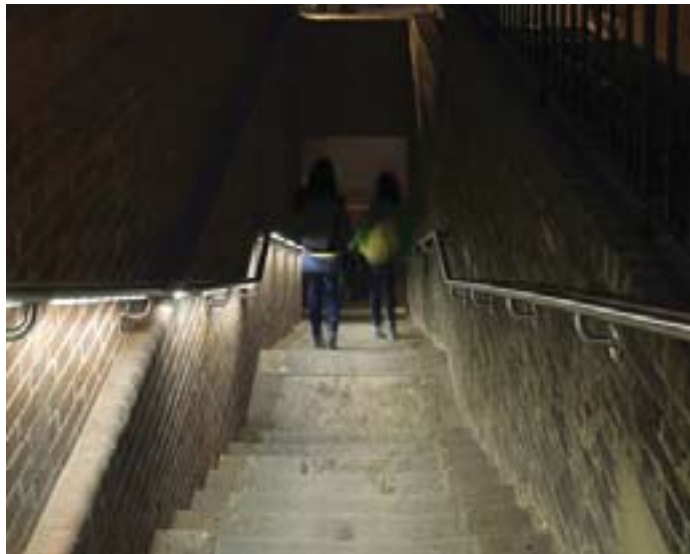
Reference images of integrated handrail lighting
