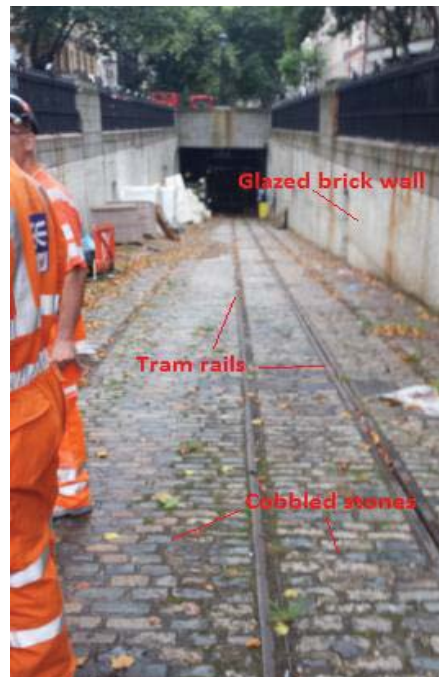
Figure 5 – KTT ramp and glazed brick walls that need protecting
