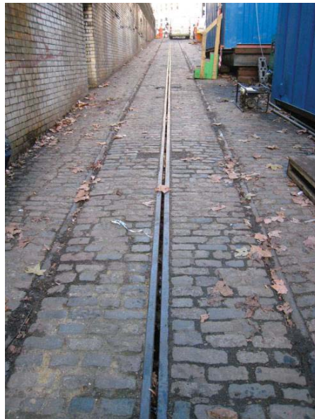
Figure 3 - Kingsway Tram tunnel entrance ramp facing North
