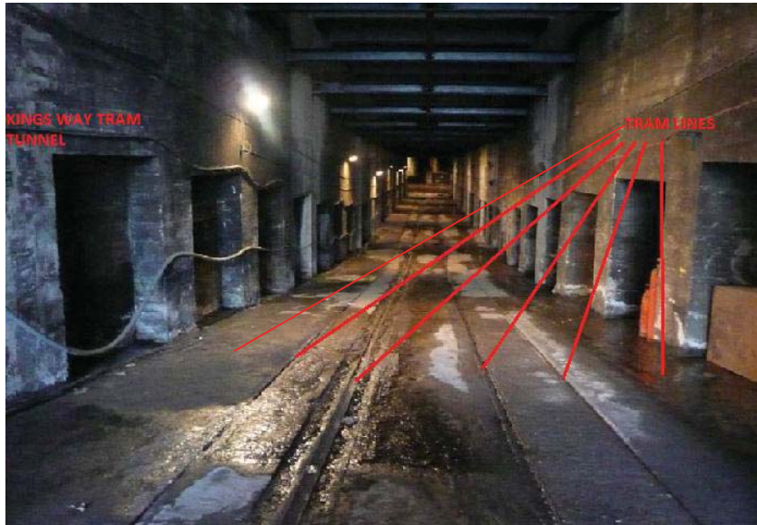
Figure 5 - Kingsway tram tunnel
