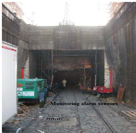
Figure 4 - Kingsway Tram tunnel entrance portal
