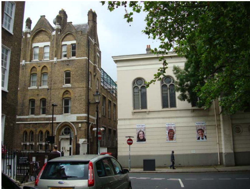
Photograph 1: East Elevation of Saint George's Church showing side windows
