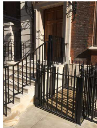
Besokpe platform lift to match railing
