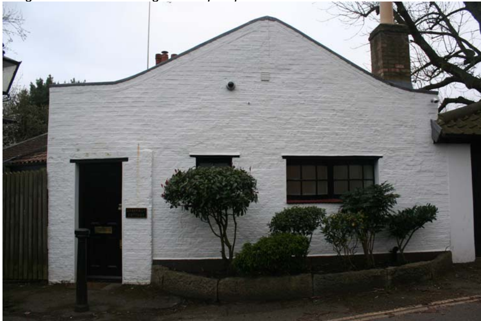
Image 6: An external image of the parapet
