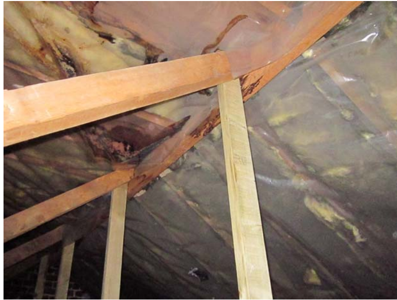
Photograph 2 – Modern softwood roof structure and plastic sheeting.
