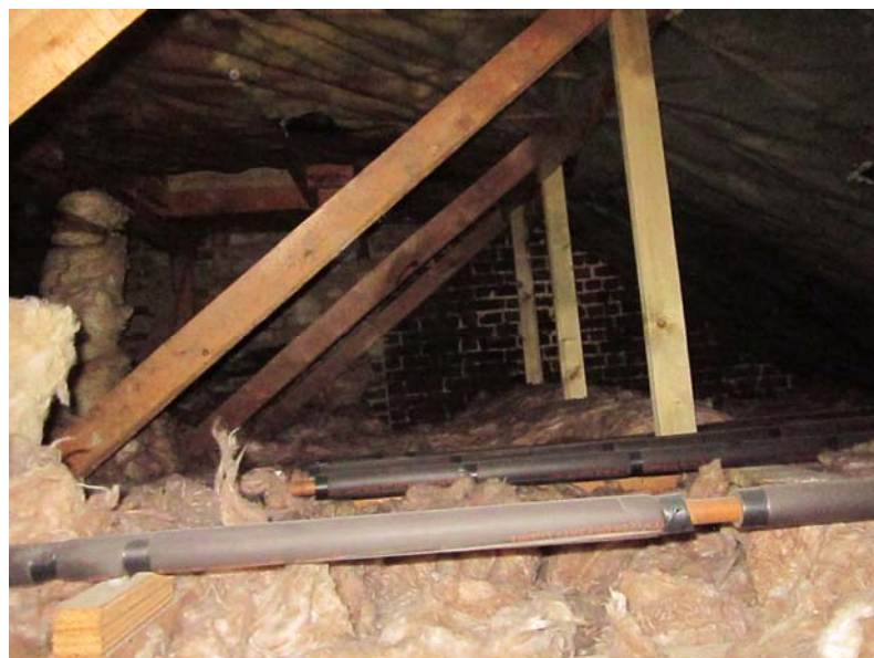
Photograph 1 – Modern softwood roof structure.
