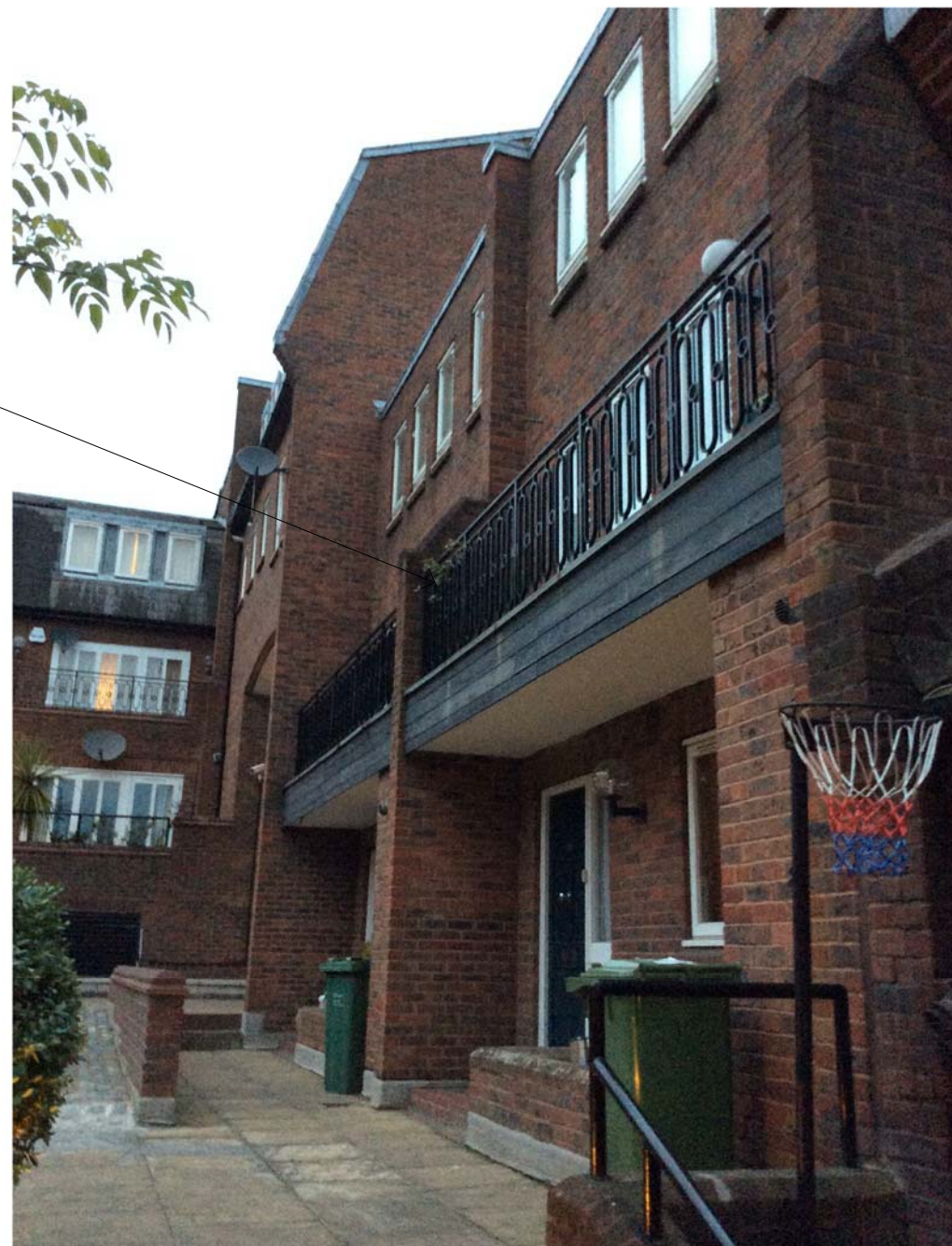
3 Timber floor balcony with metal hand
