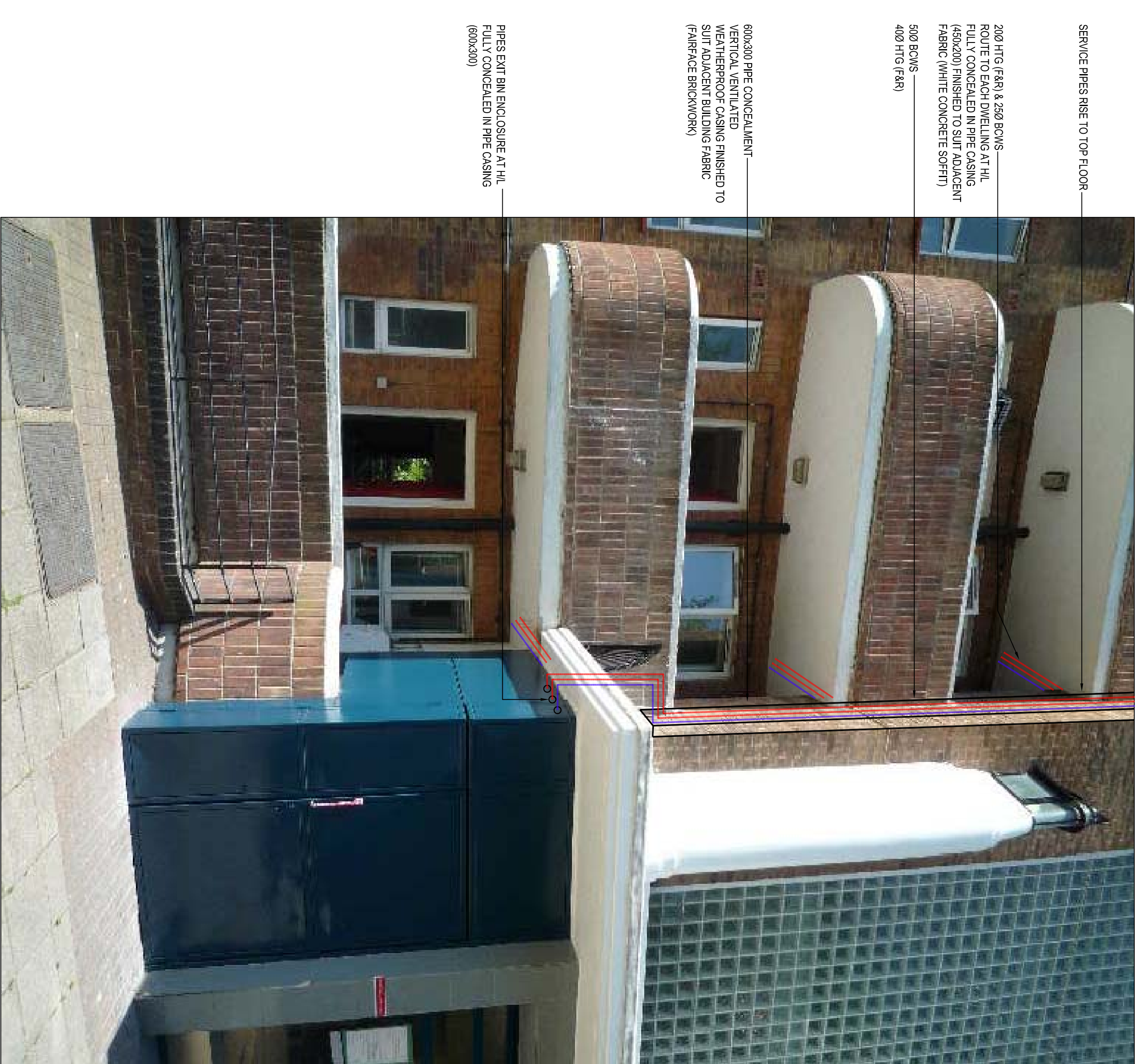
GOLDINGTON ESTATE PROPOSED SERVICES PIPE CONCEALMENT LEFT HAND SIDE OF COMMON STAIRWELL - TYPICAL (1:12 CELL HRODS)
