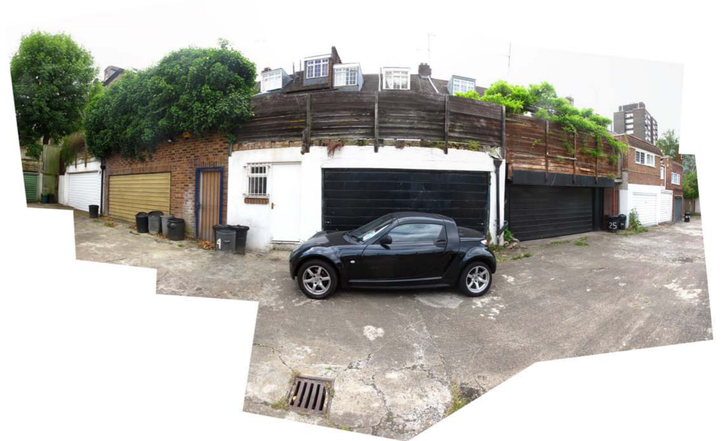
View of rear from mews accessed from Garnett Road
