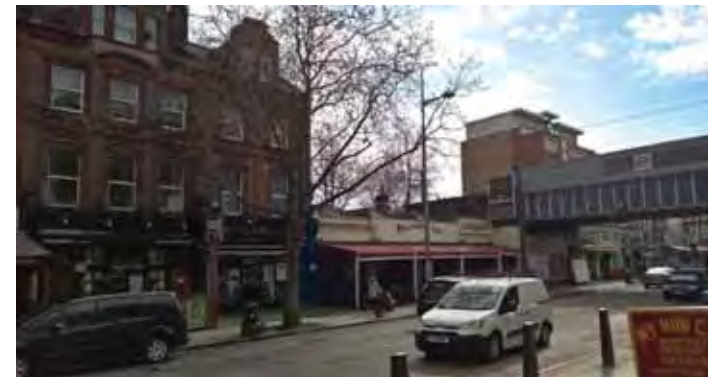
328 e-h Kilburn High Road - Existing
