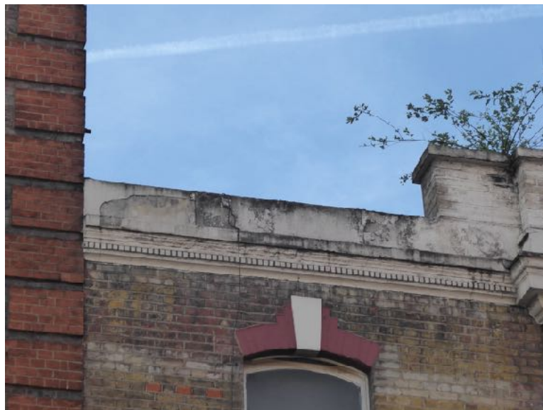
Photographs looking up at the parapet and dentil featured cornice, and second floor window head. Note the patchy historical brick repairs to the wall with red brindle bricks. Note also the smudged areas where the decorative string bands had been painted onto the brickwork.
