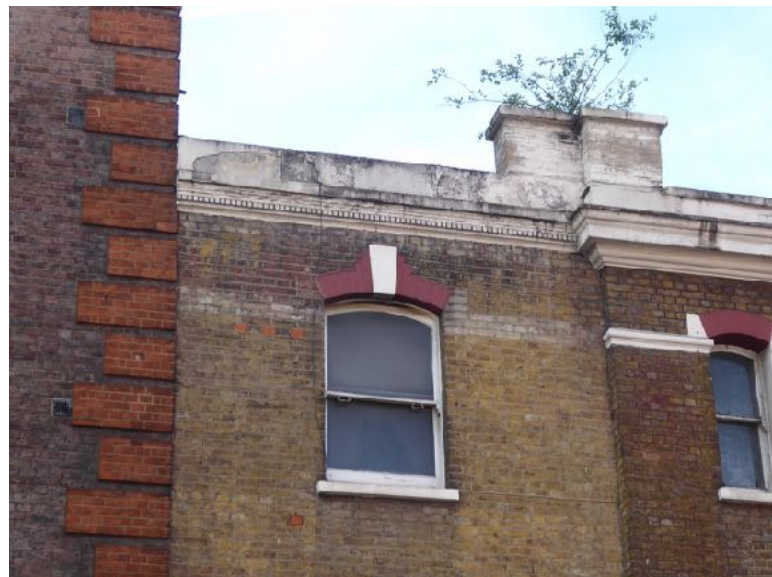
Photographs looking up at the parapet and dentil featured cornice, and second floor window head. Note the patchy historical brick repairs to the wall with red brindle bricks. Note also the smudged areas where the decorative string bands had been painted onto the brickwork.
