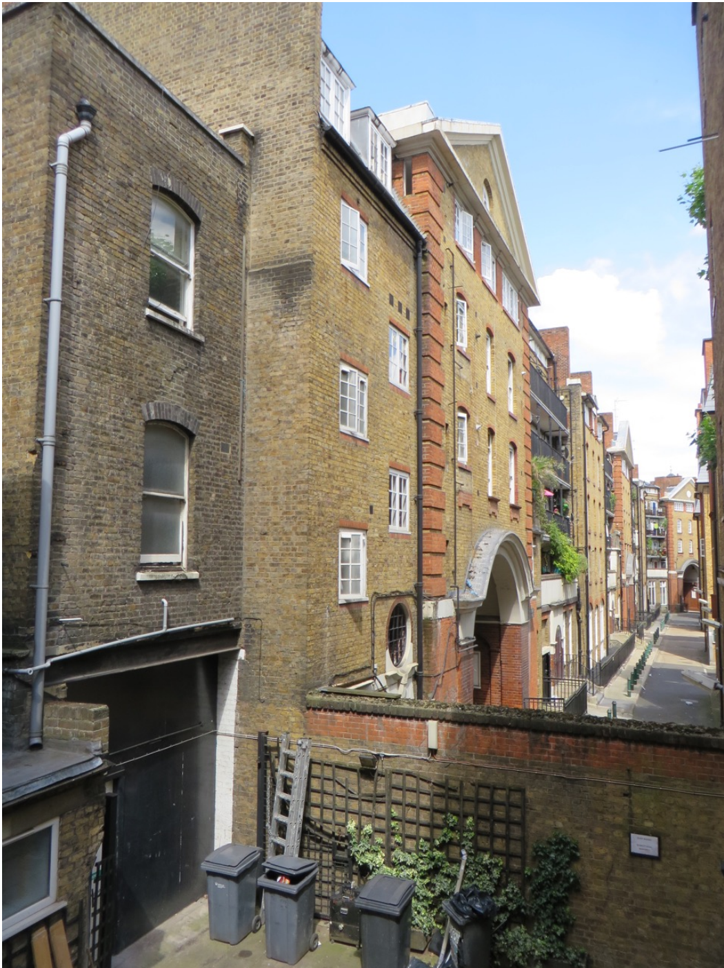
Rear view of infill element illustrating that it was built up against the flank wall of 123 Clerkenwell Road and showing the steel beam supporting the upper floors which spans onto a pad stone built into the flank wall of the adjacent property.
