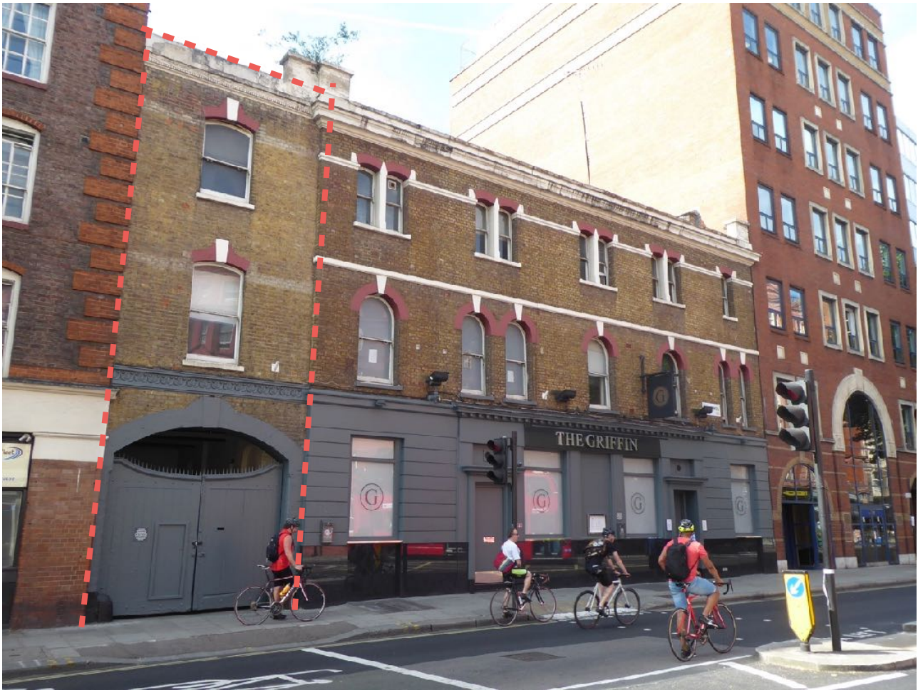
Front facade of 125 Clerkenwell Road showing the infill section in the context of the full elevation. The proposed section of the facade to be dismantled and then re-built is the eastern-most section of the elevation (within red dotted line) which is set back by half a brick.
